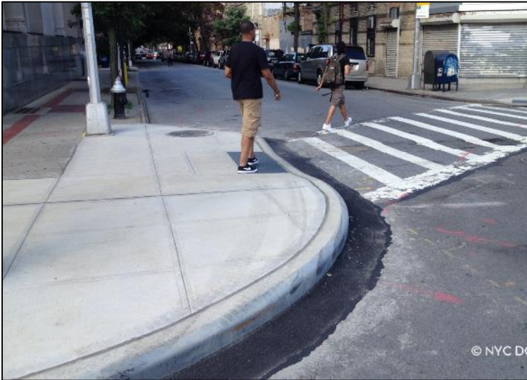
Concrete Curb Extensions
