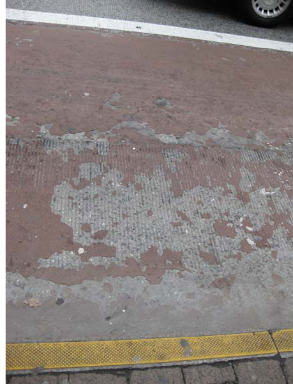
Fordham Plaza Concrete Road (Dec 2009)
