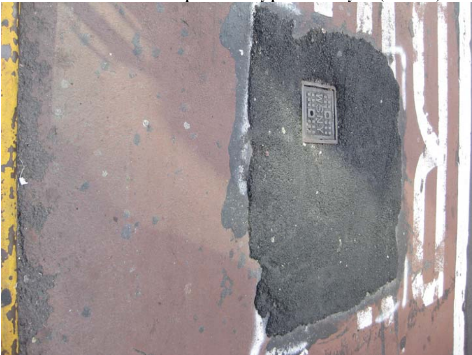
34 th Street bus lane at Harold Square – Poorly patched utility cut (Dec 2009)
