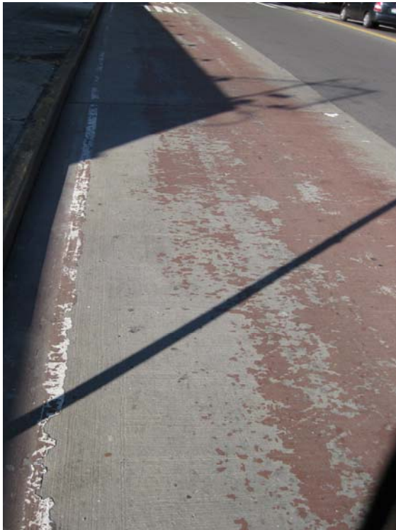
West 207 th Ave & 10 th Ave Bus Pad (Dec 2009)
