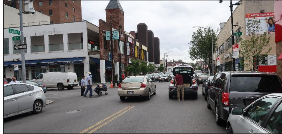
Before Conditions: Austin St at 70 th Rd
