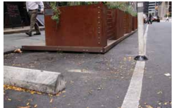
DOT will assess each site and will determine necessary traffic safety improvements.
