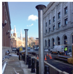
Ventilation stack
