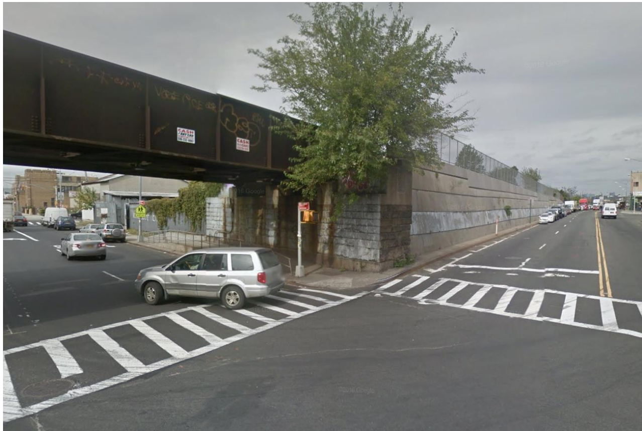
Figure 1-34 the Lower Montauk Branch Elevated on Retained Fill
