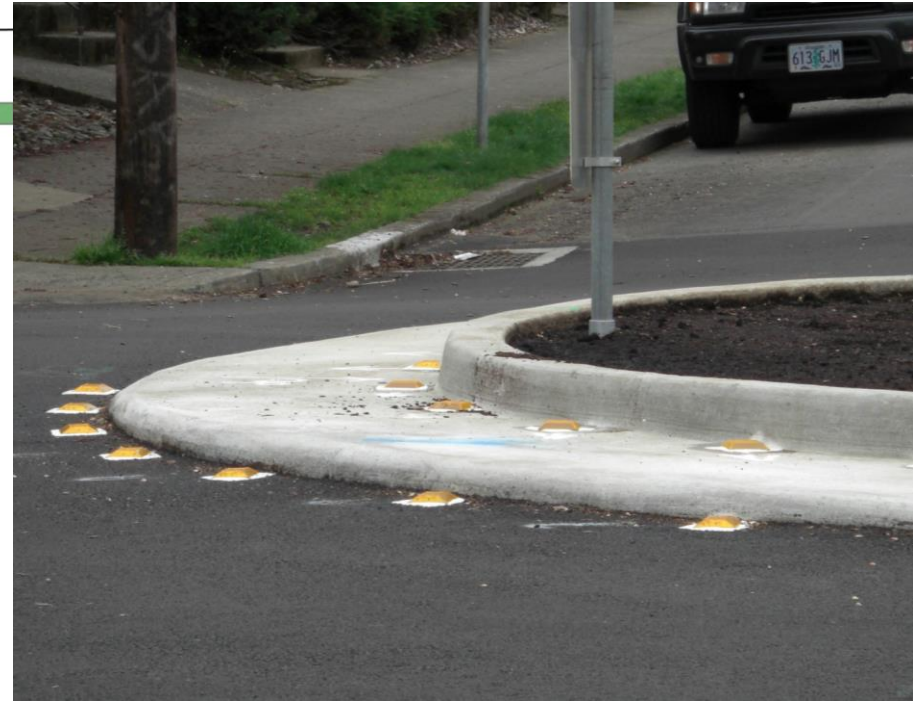
3 ft. mountable curb, Portland, OR
