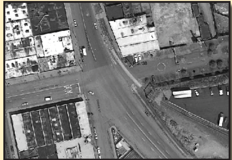
Aerial perspective of the intersection prior to improvements
