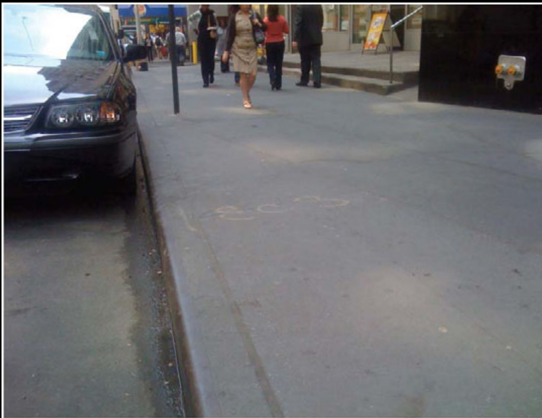
Typical tinted concrete curb with steel facing: Beaver Street at Hanover Street, Manhattan
