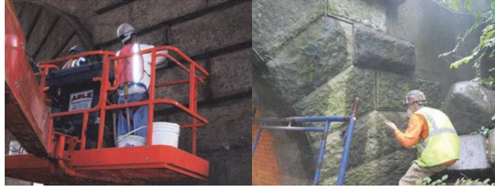
Pointing Joints on the East Face of the Brooklyn Anchorage of the Manhattan Bridge.
