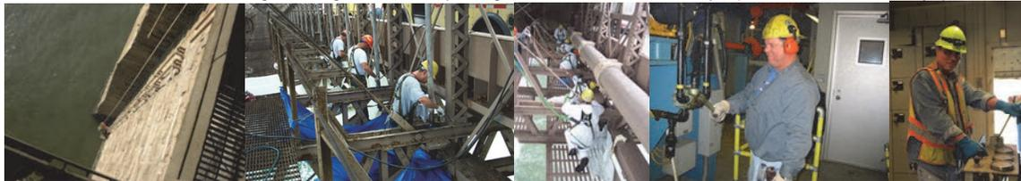
Repairing the Brooklyn Bridge Standpipe System, 130 Feet Below the Roadway. Maintenance Crew Conducting the Annual Cleaning and Lubrication of the Solid Rod Suspenders and Spherical Bearings on the Brooklyn Bridge. 2<sup>nd</sup> Photo - Oilers Steven Marxhausen, Rene Francis, Richard Morreale, Thomas McAuliffe, and Andrew Sorrentino. (Credit: Anatoly Orlov) Oiler T. McAuliffe at the 9<sup>th</sup> Street Bridge. Oiler Thomas McCarthy on the Macomb's Dam Bridge. Credit: Vera Ovetskaya)
