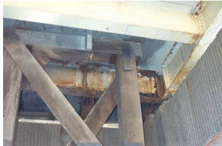
Timber Shoring Supporting a Failing Steel Beam – a Potential Winter Hazard.
