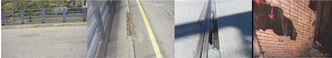
Spalled Section of Curb on the East 8<sup>th</sup> Street Bridge in 2006. (Credit: NYSDOT) Spalling With Exposed Rebar on the Beginning Abutment Joint Header of the Westchester Avenue Bridge over the Bronx River in 2011. Underdeck Spalling With Exposed Rebar on the Concourse Village Avenue Bridge over Metro North in 2012.
