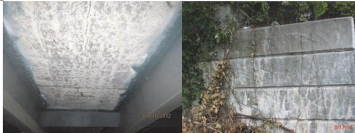
Union Street Bridge over Brooklyn-Queens Expressway in 2012 – Extensive Map Cracking With Efflorescence on the Underside of the Deck. (Credit: NYSDOT) Tompkins Avenue Bridge over B&O Railroad (Abandoned) in 2016 - Map Cracks With Efflorescence Near the End of the Wing Wall.
