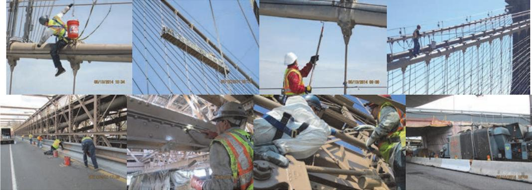
Brooklyn Bridge Contract #6 in 2014 - Painting Main Cables and Suspension Ropes. Painting at Main Bridge – Safety Barrier and Touchup. Containment at Ramp A, Span 4.
