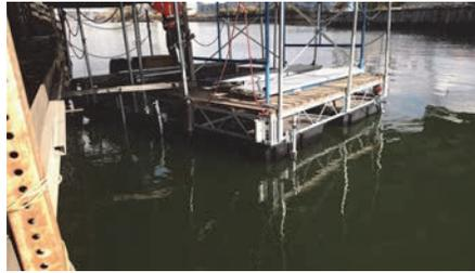
Inspector Utilizing a Motorized Platform Boat With Scaffolding to Access Most of the Underside of the Grand Street Bridge over Newtown Creek in November 2017. (Credit: NYSOT)
