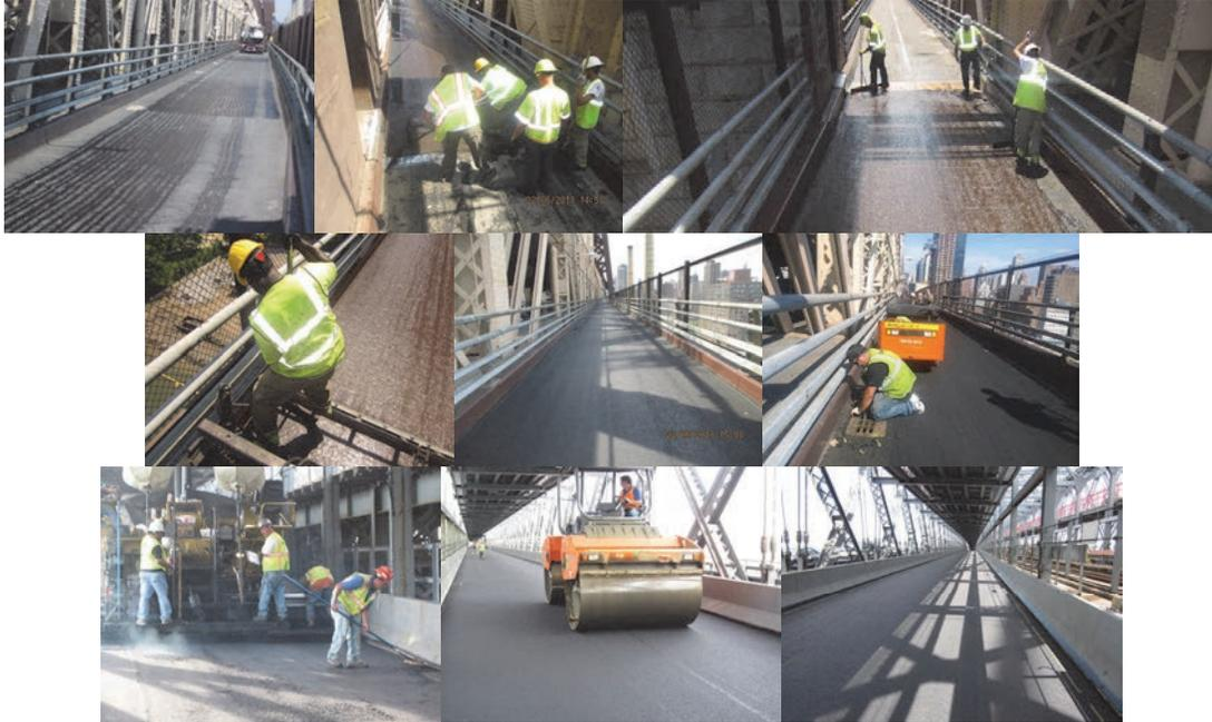
Repairing the Concrete Overlay on the South Upper Roadway of the Ed Koch – Queensboro Bridge in June 2013.
