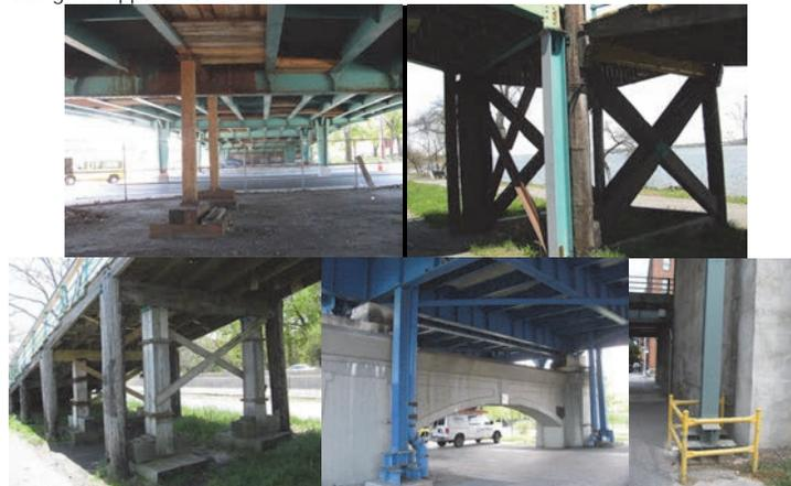
2014: Timber Shoring at Spans 7 and 8 of the Harlem River Drive over Ramp to and From Northbound Harlem River Drive. Steel Shoring of the Damaged Column at Pier 4 of the Crocheron Park Pedestrian Bridge. Timber Shoring at Piers 5 and 6. 2016: Steel Shoring at Span 5 of the East 174<sup>th</sup> Street Bridge over the Sheridan Expressway. Eastbound Brooklyn-Queens Expressway over Washington Street - Shoring on the Right Side of the End Abutment.
