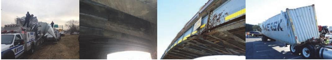
Douglaston Parkway Bridge Strike in 2015: Police Observing the Truck Damage. Underside of Bridge Concrete Beams Only Exhibited Scratches. (Credit: Artemio Angeles) 17<sup>th</sup> Avenue Pedestrian Bridge Strike in 2015.
