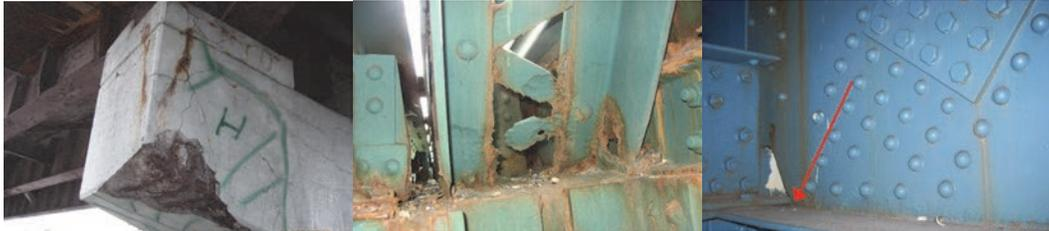
February 2008: Yellow Structural Flag Due to the Deteriorated Cap Beam. October 2008: Corrosion of Steel Secondary Member. November 2008: Crack in Steel Girder.
