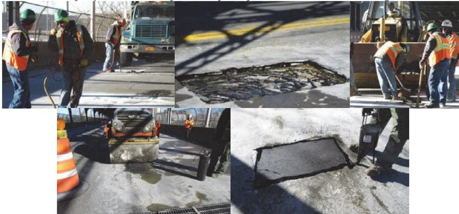
Repairing Potholes on the Roosevelt Avenue Bridge Deck Between Janet Place and 126th Street in January 2016. Each Perimeter is Sawcut. Filling in the Pothole With Asphalt. Paver Rolls Over the Pothole to Compact the Fill Material and Level the Surface. Finished Repair.
