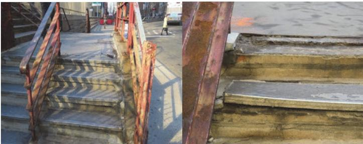
Morris Street Pedestrian Bridge in February 2017: Span #1, Near Beginning Abutment – First Step Tread Plate Missing and Second Tread Plate Broken.
