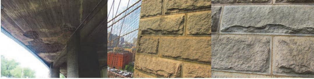
Hollow Sounding And Delaminated Concrete Areas With Exposed Rebars on the Sunrise Highway Bridge Westbound over Laurelton Parkway in 2014. Brooklyn Bridge Tower Stone Delamination in 2016.
