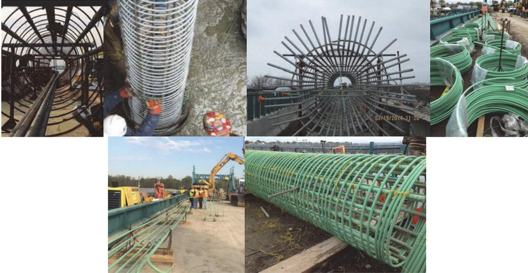
City Island, Gerittsen Inlet, and Bay Ridge Avenue Bridge Rebar Cages. 2016: Rebar Cage Assembly for the City Island Bridge. May 2016: Each Drilled Shaft Requires a Custom-Built Rebar Cage. These Steel Structures Strengthen the Concrete That is Placed Within Each Shaft Casing. Steel Bars are Laid Out on a Template to Form the Shape of the Cage, and are Then Tied Together. Once completed, the cage is Lifted by Crane and Placed Within a Corresponding Drilled Shaft.
