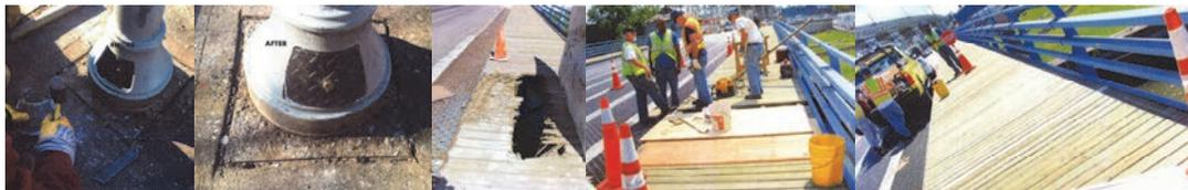
East 14<sup>th</sup> Street Bridge Over LIRR Bay Ridge –Ironworkers Fabricated and Installed the Bottom Cover of the Ventilation Post on the Right Sidewalk. June 2017 Safety Flag: Borden Avenue Bridge over Dutch Kills – Broken Wooden Planks of the Right Sidewalk at Span #1.
