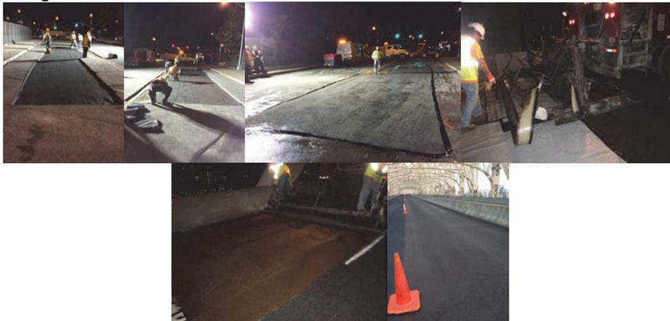
November 2014: Wearing Surface Repairs at 149<sup>th</sup> Street over the Cross Island Parkway. Applying the Waterproofing Membrane. The Finished Patch. (Credit: Steve Mezzacappa) Resurfacing the Deck of the Queens-Bound Upper Roadway of the Ed Koch - Queensboro Bridge in June 2014. (Credit: Sunil Desai)
