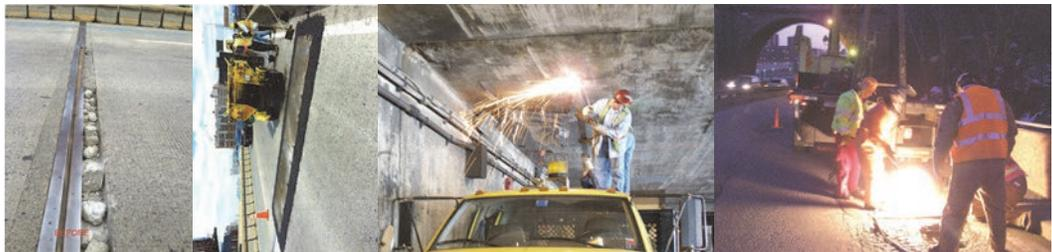
August 2014 PIA Safety Flag: Broken Joint Concrete Header And Steel Armor on the Long Island Expressway over Dutch Kills Creek. The Condition Was Made Safe By Installing Two Steel Plates. PIA Flag (Truck Wedged Under the FDR Drive at Span 41): Removing the Debris. (Credit: Victor Sandoval) PIA Flag Repair (Through Hole) on Harlem River Drive Ramp. (Credit: Bojdar Yanev)
