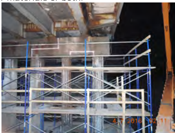
Mill Basin Bridge Scaffold Used During Pier Cap and Pier Column Repairs.
