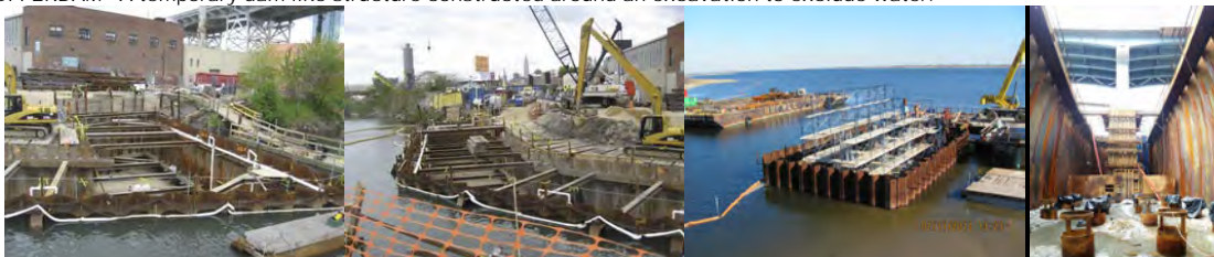
April 2010: Cofferdam With Filter Fabric and Gravel Placed Prior to Pile Driving During the Emergency Repair Project on the Borden Avenue Bridge over Dutch Kills. February 2011: Fresh Creek Bridge Cofferdam Pad. May 2016: View Inside the Gerritsen Inlet Pier 2 Cofferdam.
