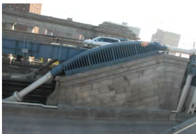
Manhattan Bridge Saddle. (Credit: Jagtar Khinda)
