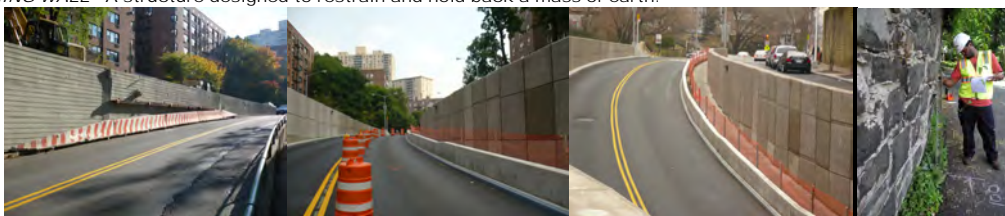
Kappock Street Retaining Wall in Riverdale, Before and After Repairs. The Existing 300-Foot Long Parallel Concrete Roadway Retaining Walls on Both Sides of Kappock Street Were Deteriorated and Leaning, and Were Replaced with New Modular Retaining Walls in the Summer of 2009. Inspecting a Bulge in a Retaining Wall Along Douglas Road in Staten Island in 2014.
