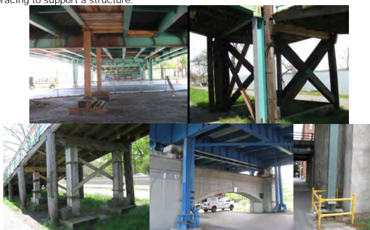
2014: Timber Shoring at Spans 7 and 8 of the Harlem River Drive over Ramp to and From Northbound Harlem River Drive. Steel Shoring of the Damaged Column at Pier 4 of the Crocheron Park Pedestrian Bridge. Timber Shoring at Piers 5 and 6. 2016: Steel Shoring at Span 5 of the East 174 th Street Bridge over the Sheridan Expressway. Eastbound Brooklyn-Queens Expressway over Washington Street – Shoring on the Right Side of the End Abutment.
