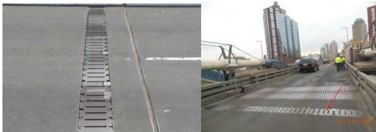
Manhattan Bridge Trench Drain.
