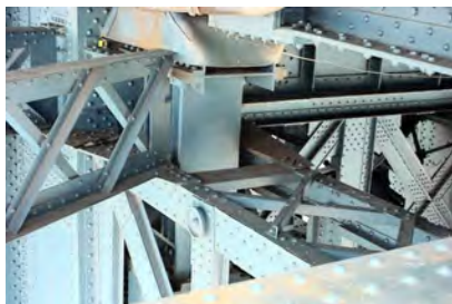
Truss Bearing on Manhattan Bridge. (Credit: NYSDOT)
