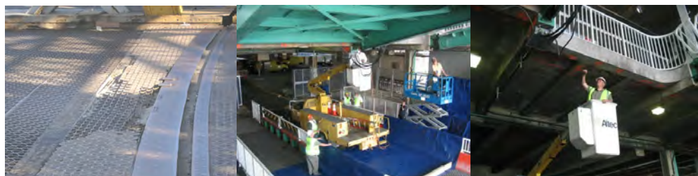
Example of PIA Safety Flag: Broken Grating. Associate Project Manager Thomas Whitehouse (White Hardhat) Ensuring the Proper Setup of Containment Procedures at the St. George Ferry Terminal Landing Slips Before the Masons Address A PIA Flag (Falling Concrete). Inspecting the Flagged Condition.
