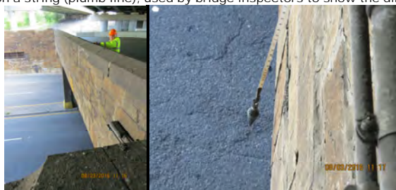
Plumb Bob in Use at Eliot Avenue Bridge over Queens Boulevard in 2016.
