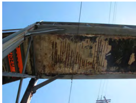
216 th Street Pedestrian Bridge in April 2016: Delaminated Concrete and Detached Exposed Rebar at Span 4 – Deck Underside.
