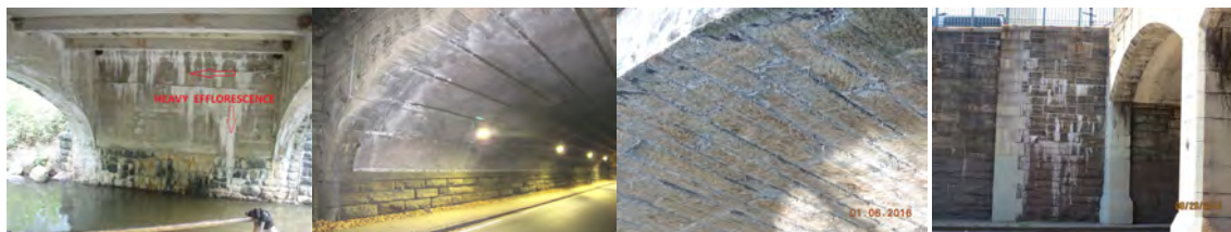
Heavy Efflorescence on End Abutment Stem Wall of Bridge Over Dam at Clove Lake in 2014. Efflorescent Stains on the Shielding of Span #1 of the East Drive Bridge over Transverse Road #3 in 2015. Efflorescence, Stalactite Formations, and Scattered Areas of Dampness and Active Water Leakage on the Underside of the Span 3 Arch of the Mosholu Parkway Bridge over the Bronx River in 2016. (Mosholu Credit: NYSDOT) Heavy Efflorescence on Cladding Stones of Crotona Avenue Bridge over Bronx Pelham Parkway in 2016.
