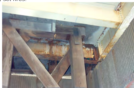
Timber Shoring Supporting a Falling Steel Beam – a Potential Winter Hazard. (Credit: Bojidar Yanev)
