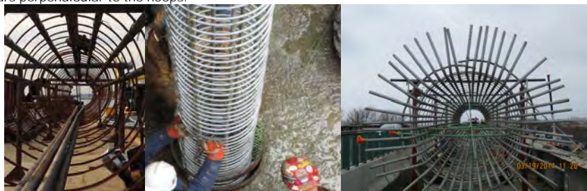
City Island, Gerittsen Inlet, and Bay Ridge Avenue Bridge Rebar Cages.
