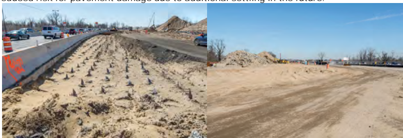
Northwest Quadrant Wick Drains for the New Mill Basin Bridge. Drains Backfilled.
