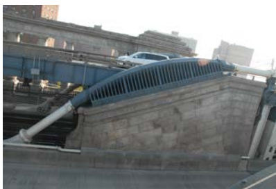
Manhattan Bridge Saddle. (Credit: Jagtar Khinda)
