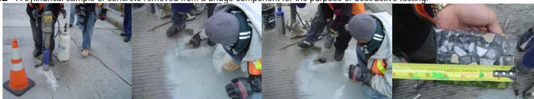
Removing a Core From 252 nd Street Bridge over Henry Hudson Parkway in January 2009. (Credit: Masroor Mahmood)
