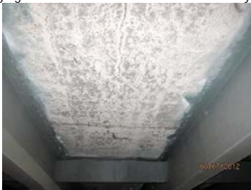
Union Street Bridge over Brooklyn-Queens Expressway in 2012 – Extensive Map Cracking With Efflorescence on the Underside of the Deck. (Credit: NYSDOT)
