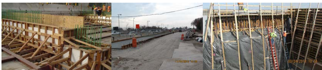
West 252 nd Street Bridge Formwork at the Pier and West Abutment in 2007. Formwork for the Westbound Roadway of the Rockaway Parkway Bridge in 2010. (Rockaway Bridge Credit: Eric Callender) Gerittsen Inlet Bridge in March 2014: Putting up Insulated Forms in Preparation for the Placement of Concrete at the West Abutment Wingwall. The Insulation Helps Protect the Concrete From the Elements and Fluctuating Temperatures During the Curing Period.
