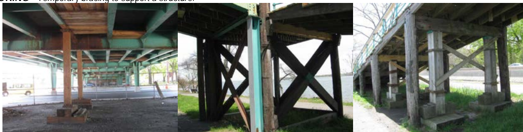
2014: Timber Shoring at Spans 7 and 8 of the Harlem River Drive over Ramp to and From Northbound Harlem River Drive. Steel Shoring of the Damaged Column at Pier 4 of the Crocheron Park Pedestrian Bridge. Timber Shoring at Piers 5 and 6.
