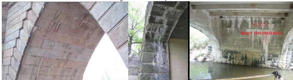
Moderate Efflorescence on the Brooklyn Bridge Brooklyn Tower North Gothic Arch in 2004. (Credit: NYSDOT) Efflorescence on the Underside of the Masonry Stones on the End Abutment of the Margaret Corbin Drive Bridge over Pedestrian Path Near Café. Heavy Efflorescence on End Abutment Stem Wall of Bridge Over Dam at Clove Lake.
