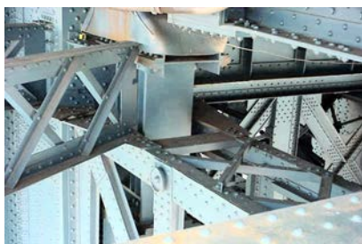
Truss Bearing on Manhattan Bridge. (Credit: NYSDOT)
