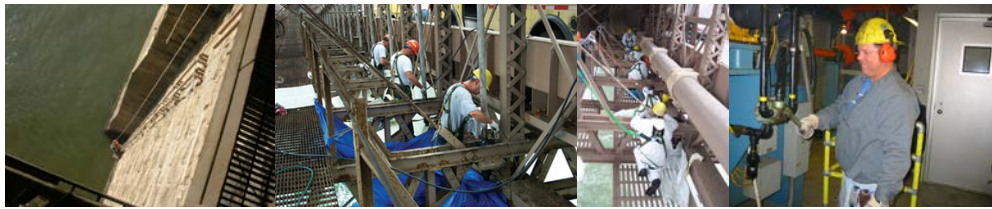
Repairing the Brooklyn Bridge Standpipe System, 130 Feet Below the Roadway. Maintenance Crew Conducting the Annual Cleaning and Lubrication of the Solid Rod Suspenders Spherical Bearings on the Brooklyn Bridge. 2 nd Photo - Oilers Steven Marxhausen, Rene Francis, Richard Morreale, Thomas McAuliffe, and Andrew Sorrentino. (Credit: Anatoly Orlov) Oiler T. McAuliffe at the 9 th Street Bridge
