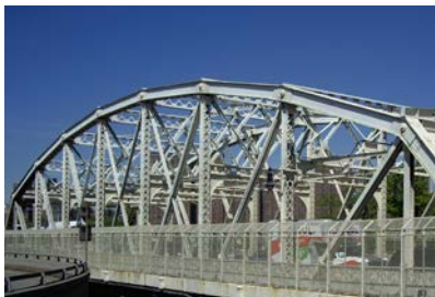
Macombs Dam Camelback Truss.
