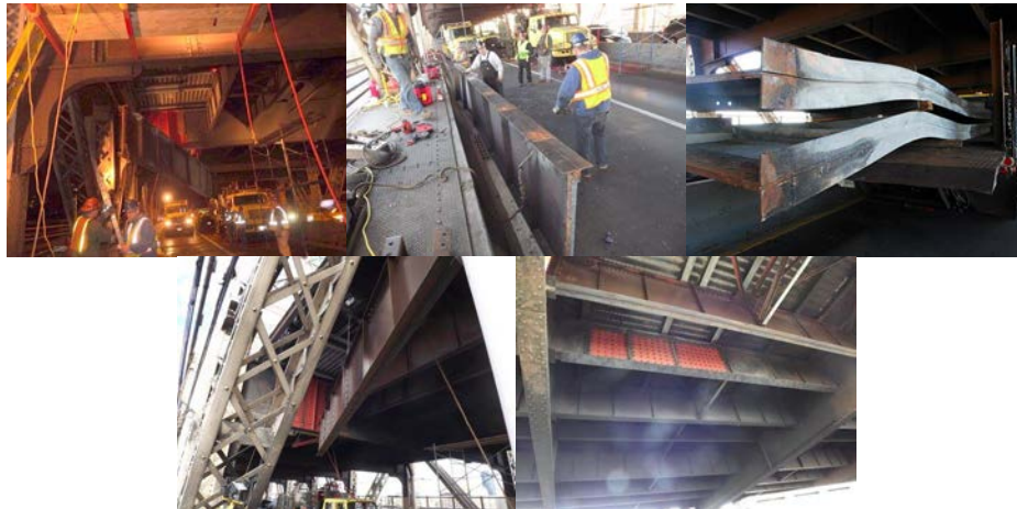
August 2013 Red Flags on the Ed Koch Queensboro Bridge. October 2013: Removing the Warped Beams. The New Beams.
