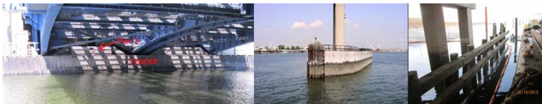
Metropolitan Avenue Bridge Fender. Rikers Island Dolphin & Fender System. (Credit: NYSDOT) Installing the Fresh Creek Bridge Fender System in 2013.
