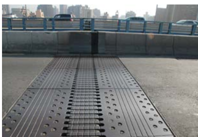
Manhattan Bridge Finger Dam. (Credit: Jagtar Khinda)
