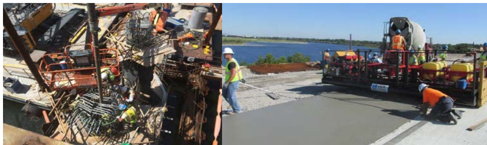
August 2014: Pumping Concrete Into Column Cage at Pier #2. Finishing Pavement at West Approach.
