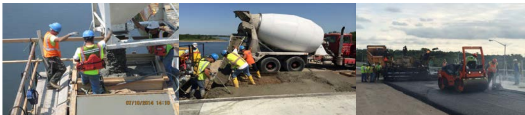
July 2014: Bottom Dump Bucket Used to Place Concrete for Pedestals at Pier #1 Cap Beam. Placing PCC Pavement at East Approach. Spreading and Compacting Hot Mix Asphalt on Belt Parkway East Side of Bridge.
