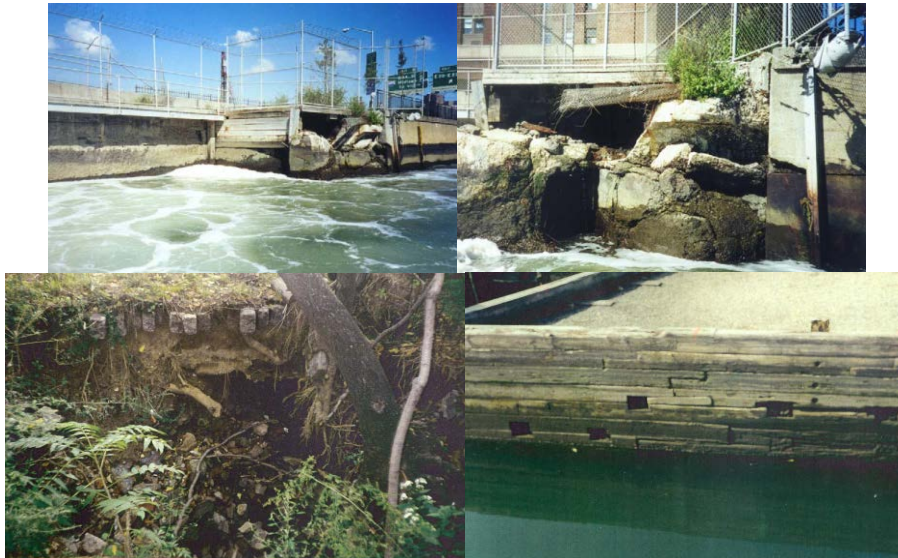
From Study of FDR Drive: Location #2 – Damaged Seawall at Segment #5. Sinkhole at Location #6 at East 59 th Street. From Study of Carroll Street Bridge: General View of the Southwest Crib Wall With the Delamination of the Timber Stretchers in the Tidal Zone.
