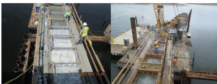
September 2014: Finishing Concrete on Pier Cap at Pier #2. Setting Forms for Concrete Pedestals at Pier #2 Cap Beam. Work Barge and Crane in Background.
