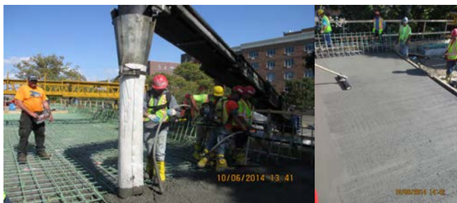
October 2014: Placing and Vibrating the Concrete Deck at the Bridge Facing West. Applying a Broom Finish Texture to the Deck Concrete.
