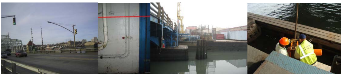
Inspection in Late 2012: East End of the West 207 th Street Bridge - Missing Traffic Signal was Knocked Down by the Hurricane Winds. Borden Avenue Bridge Operator's House Basement Level - Depicted Flood Line was Approximately 5 Feet Above the Floor. Third Street Bridge - Northwest Channel Light Missing. Ninth Street Bridge - Manually Pulling the Cable Reel Because the Motor Failed.
