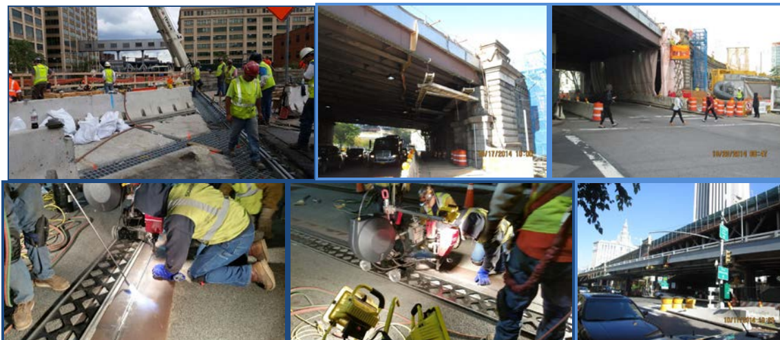
October 2014: Sands Street Structure – Preparing for Closure Pour. Containment Installation at Brooklyn Approach Structures. October 2014: Franklin Square Structure – Deck Alignment and Welding. Painted Manhattan Ramp.
