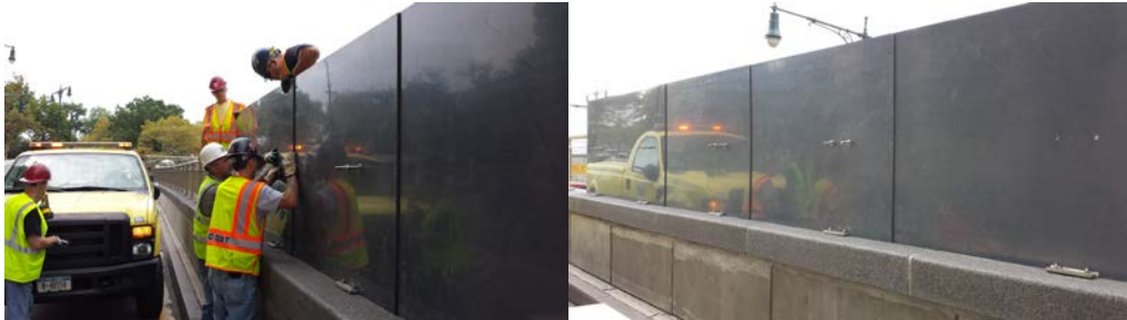
August 2014: Carpenters Stephen Buckley and William Sic, Supervisor Carpenter Joseph Vaccaro (in White Hard Hat), and Carpenters Gregory Nolan and Edward Alfano Jr. Testing the Installation of Polyvinyl Chloride Protection Boards Around the West Street Portal of the Battery Park Underpass. These Would be Placed in the Event the Coastal Storm Plan is Activated. (Credit: Paul Schwartz)
