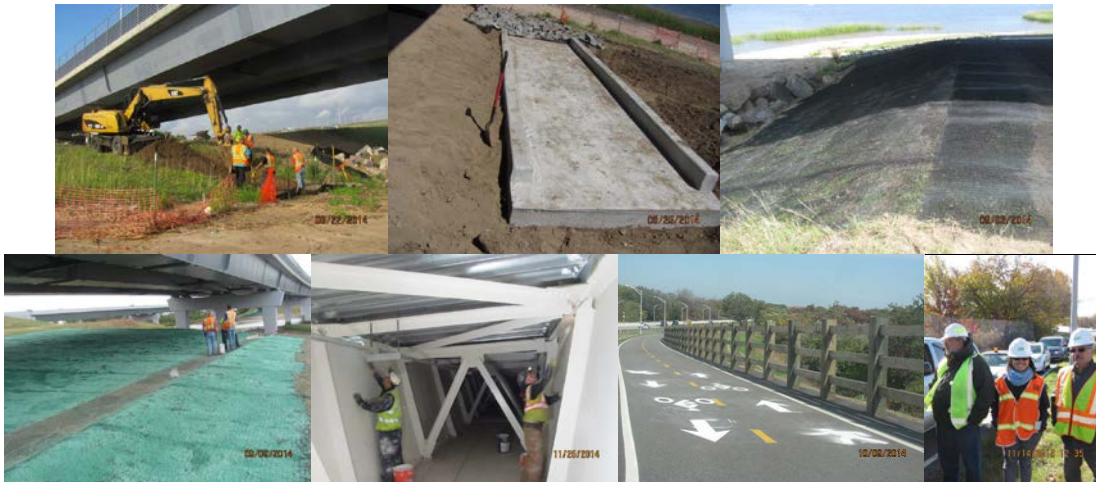
August and September 2014: Erosion Control at the Eastbound Paerdegat Bridge. Placing Fabric and Hydro-Seeding Under the Bridge. November 2014: Tub Girder Touchup Painting. October 2014: Bike Symbols on the Bicycle/Pedestrian Path East of Rockaway Circle. Three Rail Wood Fence. Associate Staff Analyst Kim Mulcahy, Civil Engineering Intern Jessica Wang, and Civil Engineer Reza Sharif at the Final Landscaping Inspection in November 2014.
