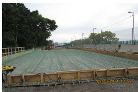
September 2014: Rebars in Place Prior to Placing Concrete Deck on Precast Concrete Beams on the North Side.
