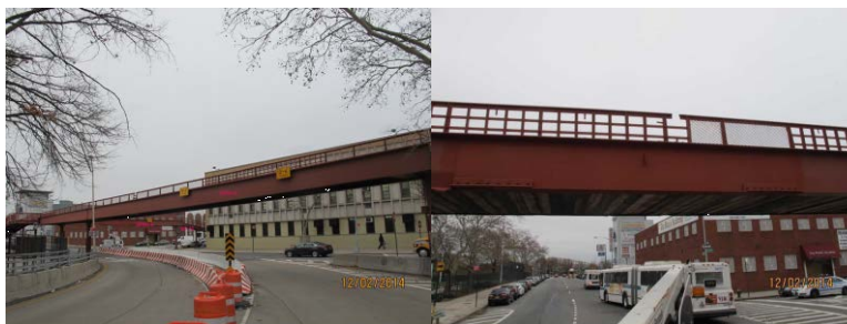
East 128 th Street Pedestrian Bridge Strike and Emergency Repairs. Left Elevation of Bridge. Timber Shielding Installed on Underside of Span #9 to Prevent Loose Concrete From Falling on the Road. Right Girder at Span #9 After Repair.
