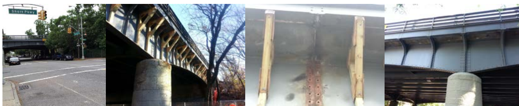
Replacing Deteriorated Fascia Brackets From the North and South Girders of the Belt Parkway Bridge Over Bedford Avenue. Temporary Supports Were Installed at the Bracket Location. Bracket was Removed. New Brackets Were Installed and Painted. (Credit: Vadim Sokolovsky)
