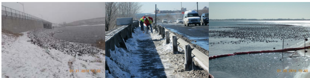
Below the Fresh Creek Bridge on January 21, 2014. Contractor Laborers Using Shovels to Remove Snow on the Pedestrian/Bicycle Path at the Gerritsen Inlet Bridge. The Path is too Narrow to Accommodate the use of Heavy Equipment. Hundreds of Ducks Gathered Near the Turbidity Curtain at the Gerritsen Inlet Bridge Project on January 29, 2014.
