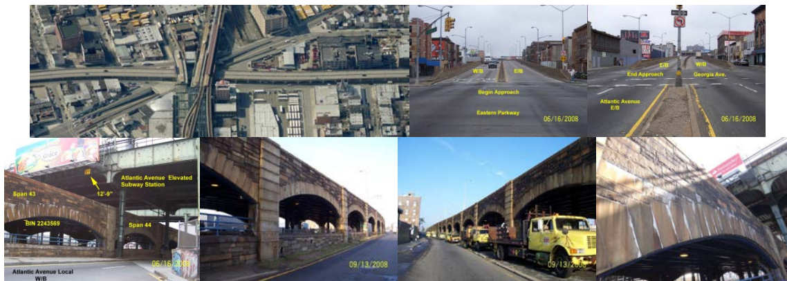
Aerial View in 2009. Beginning and End Approaches. Elevation Right – Spans 43 – 44. Elevation Left Spans 38 -43 and Elevation Right Spans 20 – 34. (Credit: NYSDOT) Span 43 South Arch Shows Typical Efflorescence at Mortar Joints of Ring Stones.
