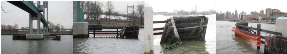
Wards Island Pedestrian Bridge – Collapsed Fender.
