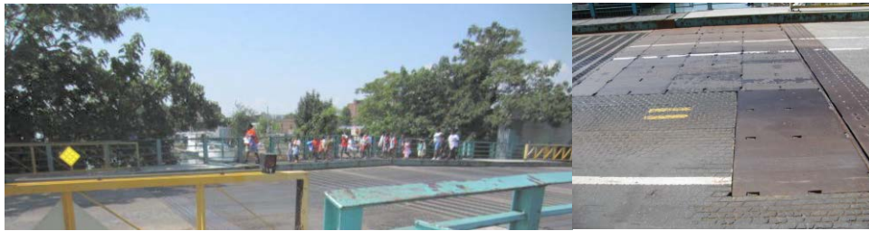
Union Street Bridge - Schoolchildren Crossing in 2012. (Credit: NYSDOT) 2014: Eleven Steel Plates Covering the Steel Grid Deck.
