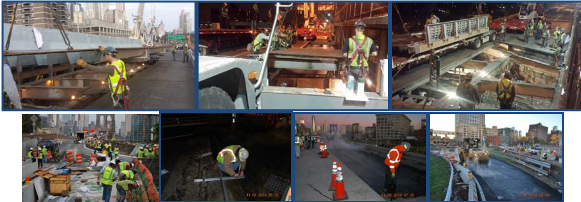
September 2014: Franklin Square Structure – New Orthotropic Deck. October 2014: Contractor Setting Rebar for Cast-in-Place Curb at Manhattan-Bound Tillary Street Access Road/Sands Street Access Road. November 2014: Manhattan-Bound Brooklyn Approach Paving.
