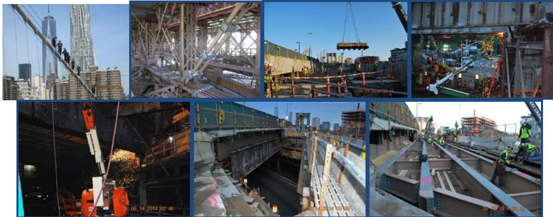
May 2014: Ascending the Cable. Installing Clamping Assemblies at the Franklin Square Structure. May 2014: Main Street Structure Westbound Overpass Replacement During Full Weekend Closure. June 2014: York Street Structure Stage II Westbound Overpass Replacement During the Full Weekend Closure.
