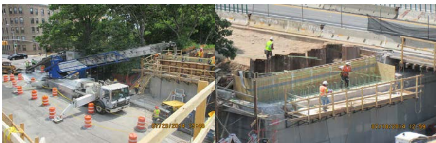
July 2014: Placing Concrete for Northeast Abutment Using a Conveyor. Setting Rebars at the Northeast Abutment.
