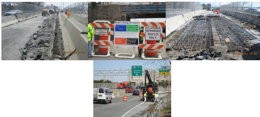
April 2014: Laborers Removing the Bridge Deck to Facilitate Removal of the Existing Concrete Median Barrier at Right Side of Trench During Stage I MPT. Stage I MPT Work Area After Removal of Structural Deck Concrete and Asphalt Wearing Courses, Exposing Deck Rebars and Structural Beams. Workers Cleaning out Catch Basins Using a High Pressure Water Hose and Vacuum Pipe for Debris Removal.
