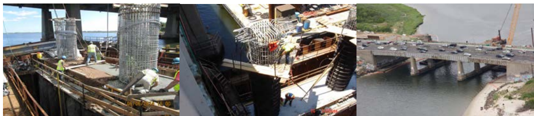
Finishing and Covering Plinth Concrete at Pier #1 in June 2014. Setting Rebars and Forms for Columns at Pier #2. Jamaica Bay at Left. Construction Barges and Cranes Constructing new Piers #1 and #2. Eastbound Traffic at Bottom.
