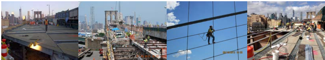
April 2014: Installation of Temporary Deck Units at the York Street Structure Over Brooklyn-Queens Expressway. July 2013: Removal of the Existing Concrete Slab on the Eastbound Main Street Structure. August 2013: Ironworker Replacing Cable Clamp Assemblies on the Suspended Span. October 2013: Grid Deck Panel Installation at the Eastbound Park Row Structure.
