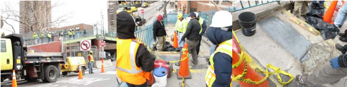
Division Staff Testing a New Patch Material on the East 25 th Street Pedestrian Bridge Over the FDR Drive in March 2014. (Credit: Bojidar Yanev)
