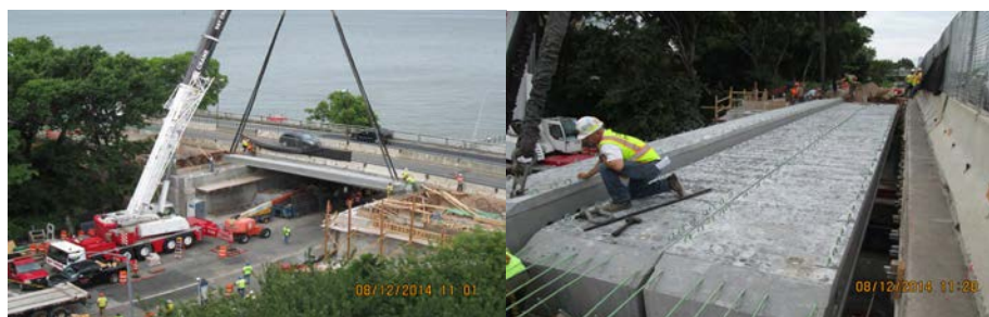
August 2014: Unloading and Placing the Pre-cast Concrete Box Beam on the North Side Abutments. Lowering the Third Pre-cast Concrete Box Beam.
