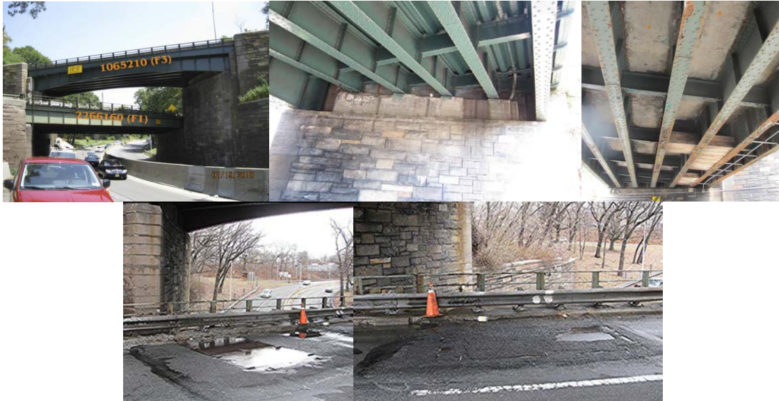
Bridge (Lower Structure) in 2010. (Credit: NYSDOT) Bridge Detail. August 2013: Span 1 Underside of Deck from End Abutment, Looking Northwest - Areas of Spalled Concrete Deck Are Protected With Timber Planks. March 2014: Steel Plates on Wearing Surface.
