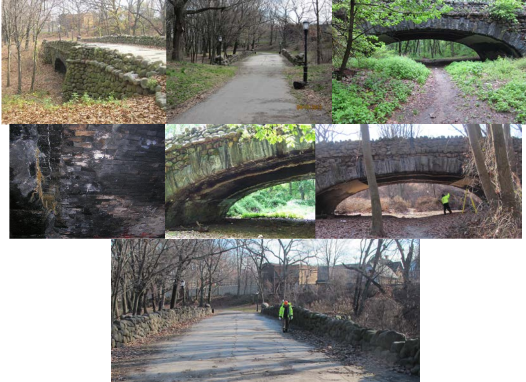
Highland Park Bridge. Dirt Pathway Under Bridge. Under-Deck Cracks and Missing Bricks - North-East Side. Under-Deck Arch Wall Showing Efflorescence Along the Cladding Stone and Brick Arch. Inspecting the Bridge in December 2014.
