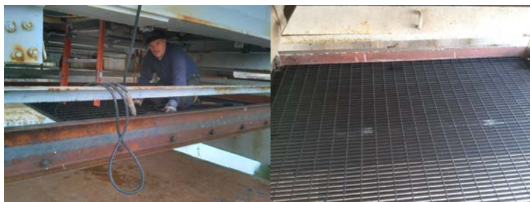
March 2014: Bridge Repairer & Riveter Daniel Jaderlinic Welding New Steel Grating and Support Framework on the Rikers Island Bridge. (Credit: Steve Havemann)
