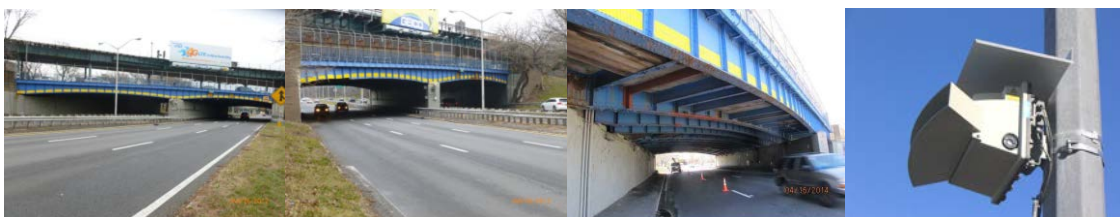
Westchester Avenue Bridge Elevation Left and Right in 2012. (Credit: NYSDOT) April 2014: Span 2 – Deteriorated Areas Shielded With Planks. Overheight Sensor Unit on the Hutchinson River Parkway. (Sensor Credit: Roly Parroco)
