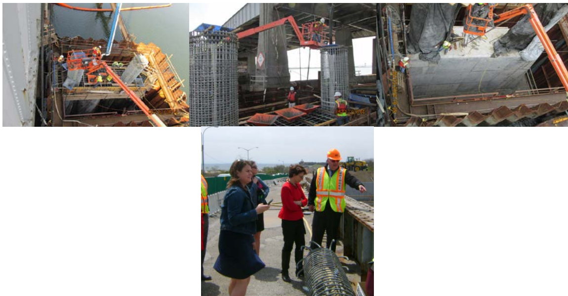
Pier 1 Plinth and Footing Inside the Cofferdam in May 2014. Commissioner Polly Trottenberg (in Red Jacket) and Chief Bridge Officer Robert O. Collyer Inspecting the Gerritsen Inlet Bridge Project in May 2014. (Credit: Moshin Rizvi)
