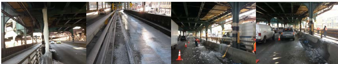
Huge Icicle (Caused by a Broken Water Pipe) Between the South Outer Roadway and the Inner Roadway at the Queens Approach of the Ed Koch – Queensboro Bridge. Icing on the South Outer Roadway. Division Engineers Closed Parts of the Roadway Until NYCTA Crews Completed the Removal of the Icicle and All of the Ice From the Roadway Surface and Barrier. Salt was Placed on the Remaining Ice on the Roadway. (Credit: Artemio Angeles)
