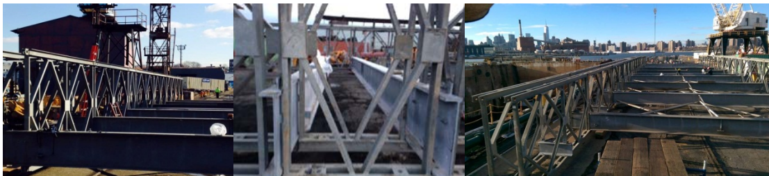
The Contractor Assembled the Temporary Bridge Segments at the Brooklyn Navy Yard. The Pieces Were Transported to City Island by Barge.
