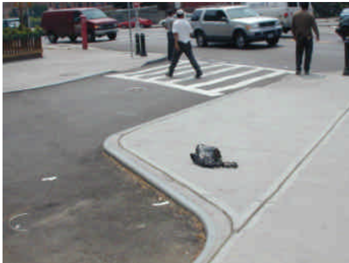
Figure 6.14 Gateway treatment at Fulton Street and South Oxford Street
