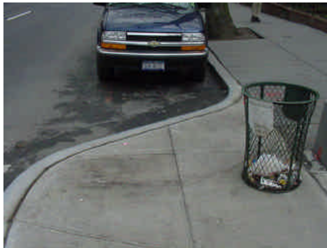
Figure 6.21 Lafayette Avenue neckdown: Small curb radius created areas difficult to reach with streetsweepers
