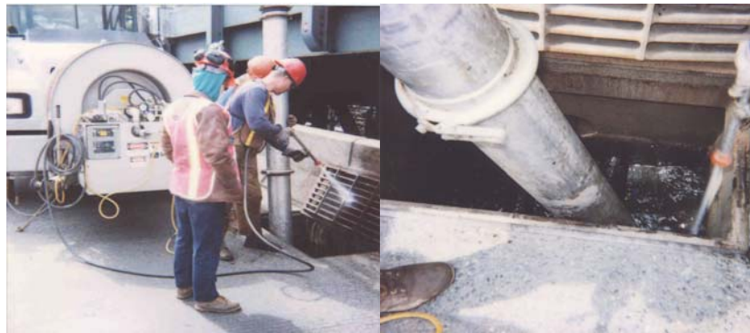
Cleaning Catch Basins on the Manhattan Bridge.
