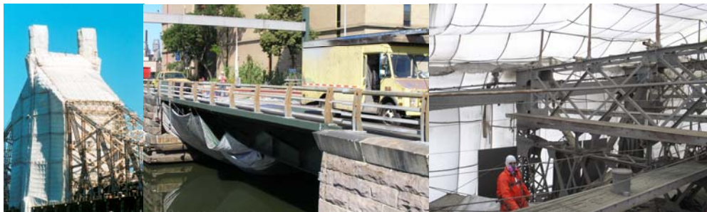
2005: Queensboro Bridge Containment. (Credit: Peter Basich) 2005: Preventing Paint From Falling Into the Dutch Kills under the Hunters Point Avenue Bridge. (Credit: Sergiy Parayev) Working Inside the Queensboro Bridge Containment.
