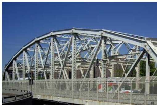
Macombs Dam Camelback Truss.
