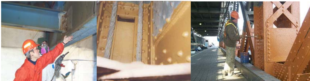
Spot Cleaning Before Painting on the Williamsburg Bridge. Primer Coating on the Williamsburg Bridge. Salt Splash Painting on the Williamsburg Bridge. (Salt Splash Credit: Fouad Althaibani)
