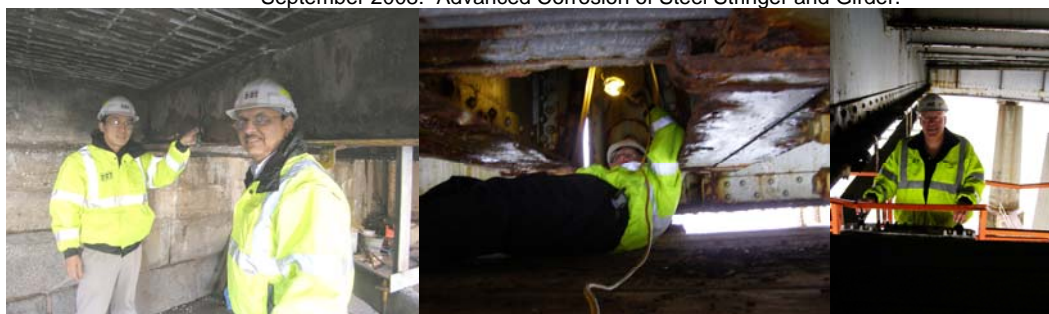
Assistant Civil Engineer Andrew Hoang and Civil Engineer Rajendra Pandya Measuring the Section Loss of the Bottom Flange of A Floor Beam, Utilizing a Digital Caliper. Executive Director of Bridge Preventive Maintenance and Repair Thomas Whitehouse Inspecting a Red Flag on a Girder Floor Beam at the Belt Parkway Bridge over Gerritsen Inlet. Mr. Whitehouse Operating a Zoomboom. (Gerritsen Credit: Steve Havemann)
