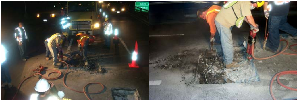
Masonry Crews and Highway Repairers Repairing Recurrent Potholes on the Eastbound Brooklyn-Queens Expressway, Just Past the Middagh Street Underpass. Break-Out and Removal of the Old Asphalt Roadway and Concrete Deck. (Credit: Anthony Napolitano)
