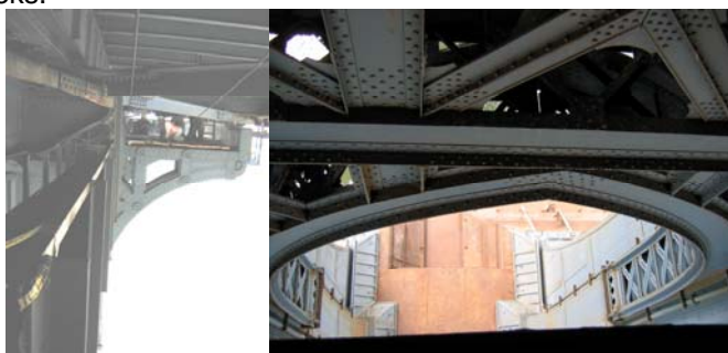
Flag Engineers Inspecting a Red Flag (Floor Beam Web) on the Tower Structure of the Manhattan Bridge. Closeup of the Location. (Credit: Bojidar Yanev)
