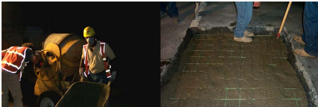
Installing New Concrete With Rebar in the Cutout on the Eastbound BQE. (Credit: Anthony Napolitano)
