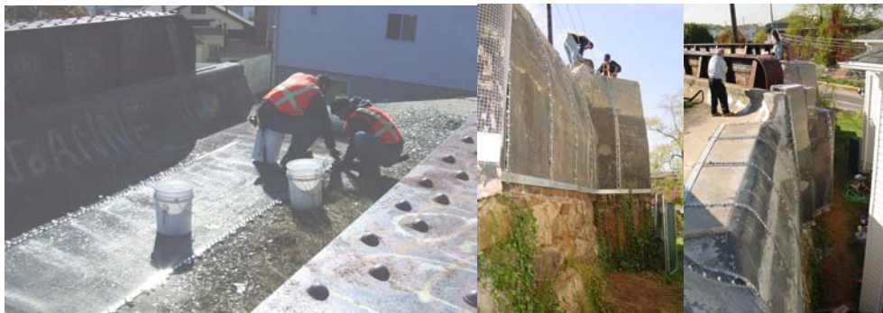
An Emergency Safety Netting System was Installed at Both Ends of the Abutment of the Abandoned Railroad Bridge Over Robin Road to Protect the Adjoining Property Owners From Falling Deteriorated Concrete. (Credit: Thomas Leung)
