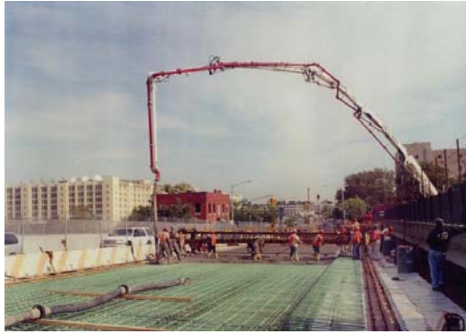
Placing the Deck Concrete.
