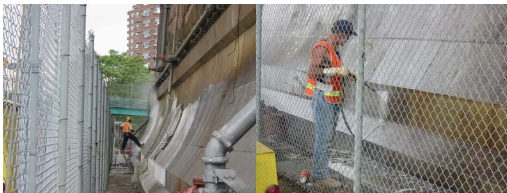
Removing Graffiti From the Manhattan Pier of the Williamsburg Bridge. (Credit: Vadim Sokolovsky)
