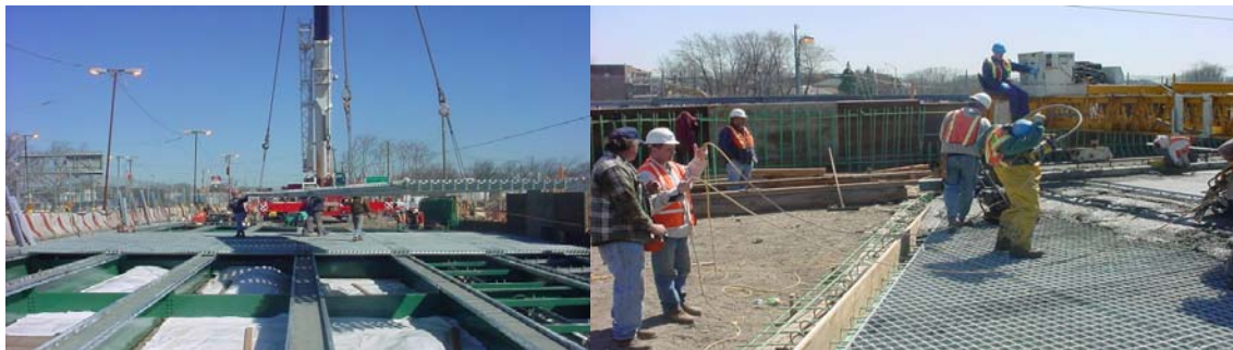
Placement of the Grid Deck Panels. Placing the Concrete for the Grid Deck. (Credit: Muhammad Siddiqui)
