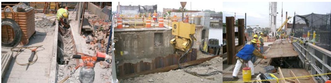
Demolition of the Northwest Flanking Span of the Metropolitan Avenue Bridge. Looking West at the Installation of Sheet Piles on the Northeast Approach Slab. Looking West at the Removal of the Northwest Sidewalk.
