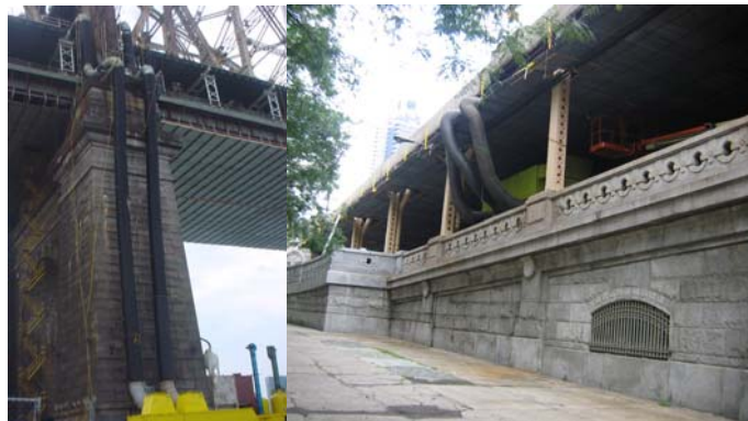
Work Platform and Containment Installation on the Queensboro Bridge. (Credit: Daniel Lima) Painting in Progress on the South Outer Roadway. (Credit: Peter Basich)
