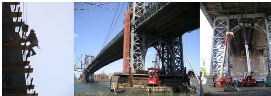
Strengthening Plate Operation on Brooklyn Main Tower. Pier Stationed & Barge Mounted Cranes at Brooklyn Main Tower Pier. Steel Arch Replacement.
