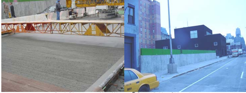
Deck Placement. New West 37 th Street Bridge Sidewalk.
