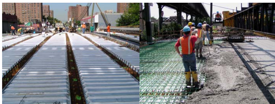
Installing Stay-in-Place Forms on the Sutter Avenue Bridge. Placing the Bridge Deck Concrete.
