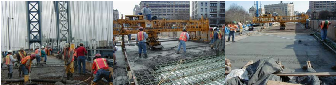
Contract #10 Placing Concrete on the Manhattan Side Span Grid Deck of the North Upper Roadway. Placing and Finishing Concrete on the Grid Deck of the Brooklyn Elevated Structure.
