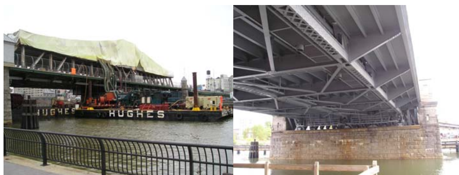
Madison Avenue Bridge Containment. Detail of Freshly Painted Bridge.
