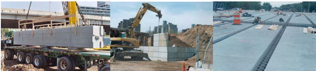
Precast Pier Capbeam Section Prior to Setting it on the Cast-in-Place Columns. Installing T-Walls. Precast Panels and Joints Awaiting Cast-in-Place Concrete Placement.
