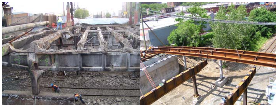
Demolishing the Old Sutter Avenue Bridge. Erecting Structural Steel.
