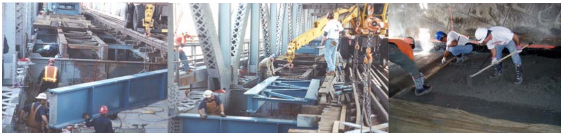
Contract #10 Installation of New Floorbeams & Stringer Panels for the Subway Support Steel. Placing the Waterproof Protection Layer on the Anchorage Roof Inside the North Track Envelope.
