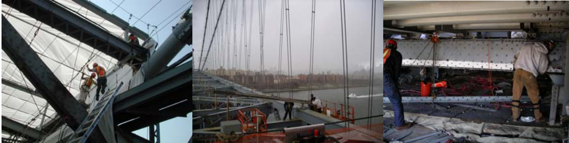
Contract #8 North Stiffening Truss Containment Erection and Removal. South Truss Bottom Chord Rehabilitation.
