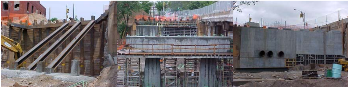
Excavation Protection System at the New 2 nd Avenue Bridge North Abutment. View of the Partially Completed Center Pier and South Abutment. View of the New North Abutment Stem Wall.
