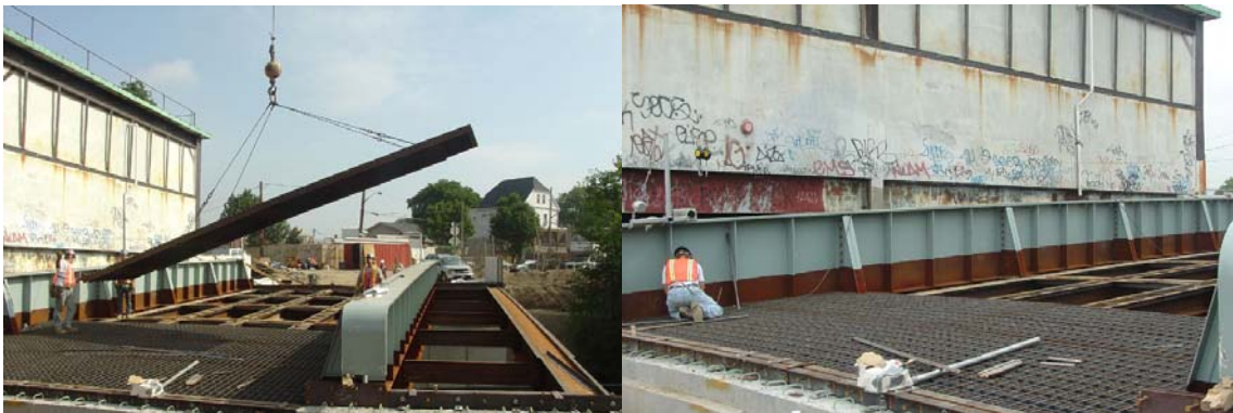
Installation of the Grid Deck on the New Andrews Avenue Bridge.
