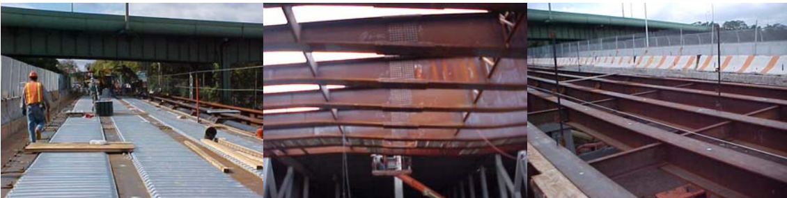
Installation of Stay-in-Place Deck Forms on the 2 nd Avenue Bridge. Structural Steel Erection.
