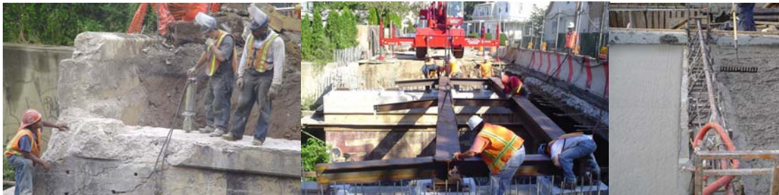
Demolition of the East 3 rd Street Bridge South Abutment. Installing Structural Steel. Placing Concrete for the Approach Slabs.
