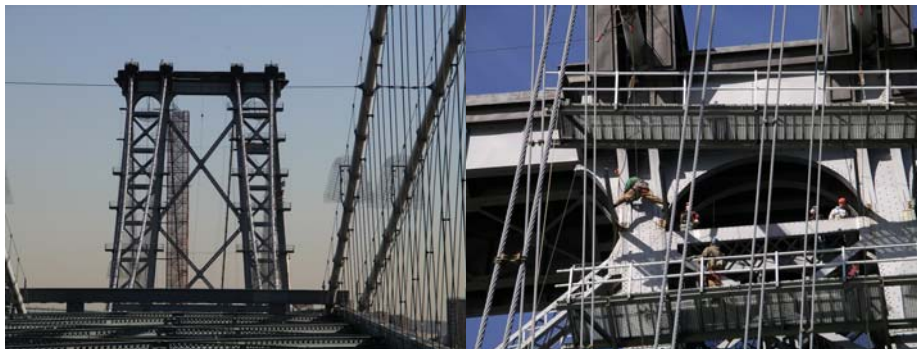
Contract #8. Looking East at the Brooklyn Main Tower Temporary Work Platforms. Manhattan Main Tower Temporary Platform Erection.
