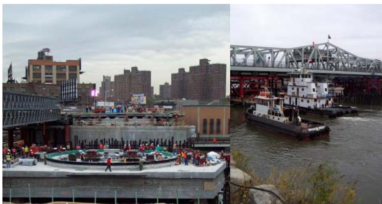
Preparing for the Float-in of the New Swing Span. Tugboats Pushing the Span Into Final Position. (Credit: Keith Burrowes)
