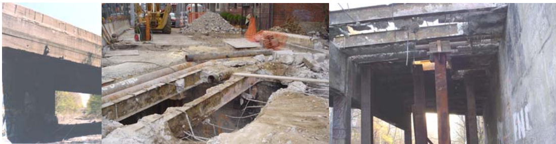
52 nd Street Bridge Before Reconstruction. Demolition of the Bridge Deck. Installation of Temporary Supports.
