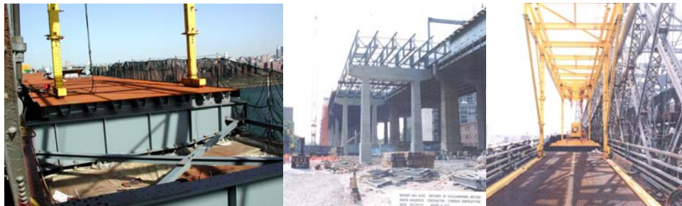
Contract #7 Installing An Orthotropic Deck Panel. Working on the North Roadways.
