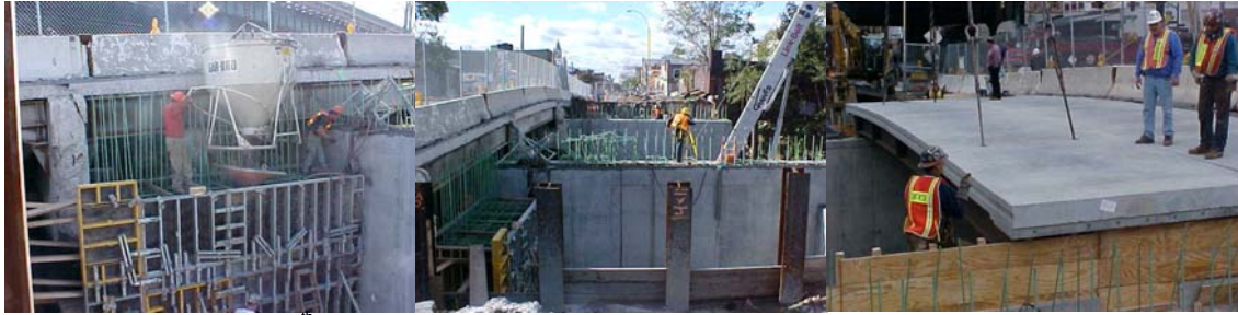
Concrete Pour at the 14 th Avenue Bridge Abutment. View of the Partially Completed Abutments. Installing the Precast Panels.
