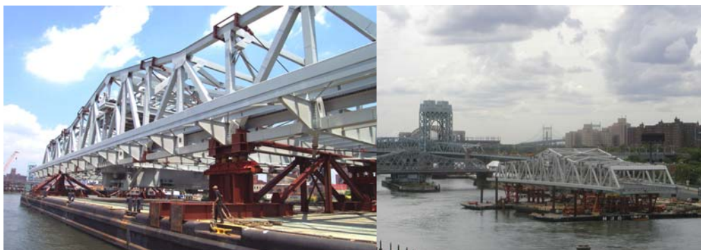
Ocean Barge Arrival at the Bridge Site. (Credit: Bojidar Yanev) New Swing Span on the Working Barges. (Credit: Daniel Hom)
