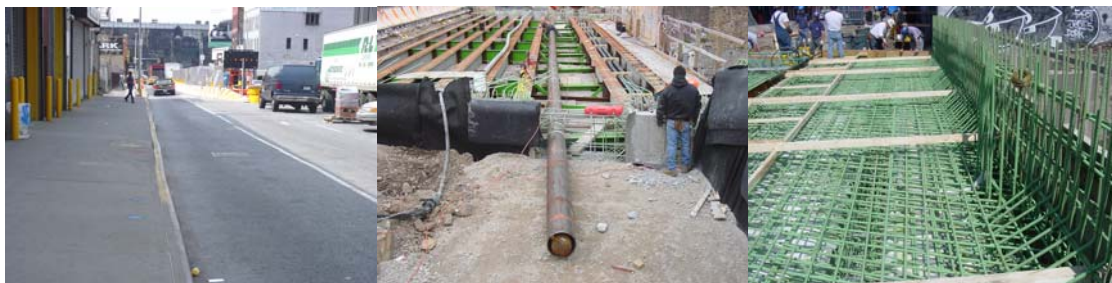
West 37 th Street Bridge Before Reconstruction. Stage 1 Construction. Deck Pour.
