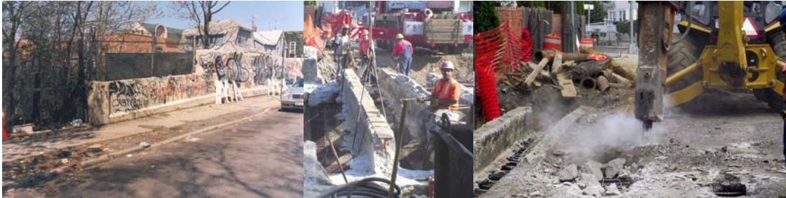
East 3 rd Street Bridge Before Reconstruction. Removing the Stringer Encasements. Removing the West Side Bridge Deck.
