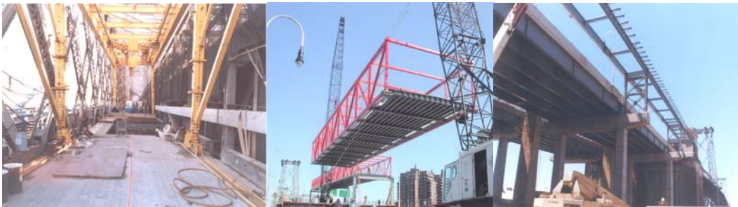
Contract #7 Replacing the North Inner Roadway Deck & Erecting the Footwalk. Bikeway Steel Erection.
