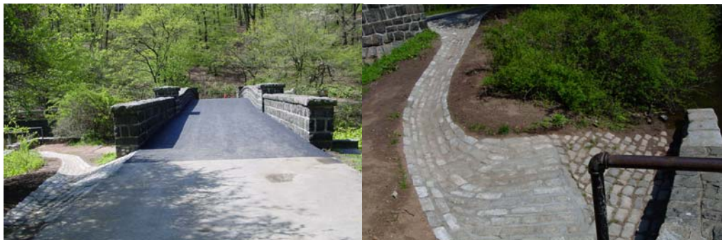
Bridge over Dam at North End of Clove Lake—the Deteriorated Asphalt Wearing Surface was Restored & a New Belgian Block Drainage Trough System was Installed. (Credit: Thomas Leung)
