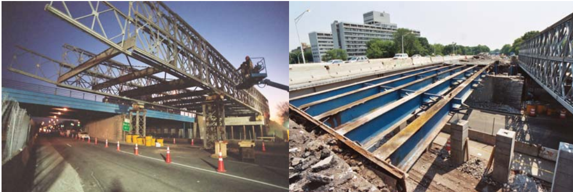
Launching of the 54 Meter (190 ft) Temporary Bridge in February 2004. Original Bridge Under Demolition.
