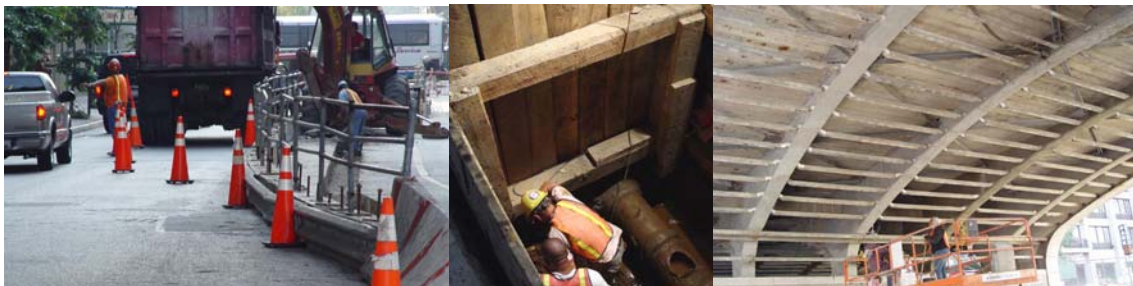
Starting Curb Replacement at 60 th Street. Improving the Drains at the Vehicle Storage Area. Repairing Spalled Concrete at the 59th Street Overpass.
