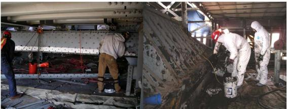
Contract #8 South Truss Bottom Chord Rehabilitation. .Degreasing the Brooklyn Main Tower Saddle Bearing.
