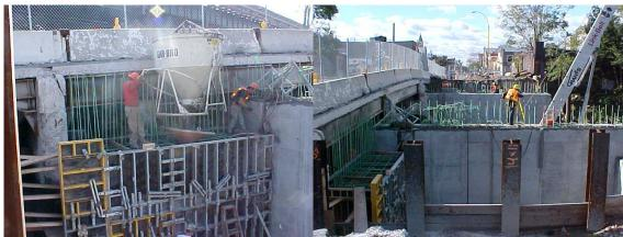
Concrete Pour at the 14<sup>th</sup> Avenue Bridge Abutment. View of the Partially Completed Abutments.
