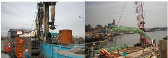
Auger Excavation of the Drilled Shaft at the Third Avenue Bridge Manhattan Rest Pier From the existing Bridge Deck.
