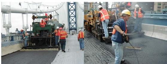
Placing the Microsurfacing Overlay on the Main Span. Placing the Asphalt Overlay on the Brooklyn Approach Span.
