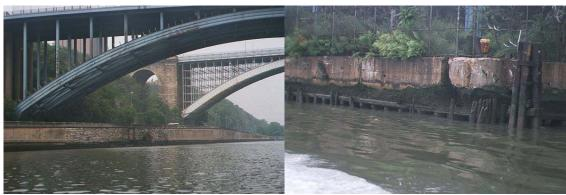
Bulkhead at Alexander Hamilton Bridge. Severe Erosion of the Concrete Seawall Allowing Loss of Fill at the MTA Rail Yard at 151<sup>st</sup> Street.
