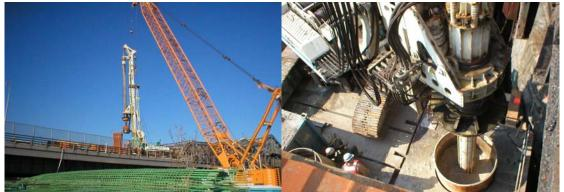
Drill Rig Installing the Third Avenue Bridge Manhattan Rest Pier Shaft from the Existing Bridge Deck. The Rebar Assembly and Staging Area are in the Foreground. Drill Rig Excavating the Drilled Shaft at the Center Pivot Pier.
