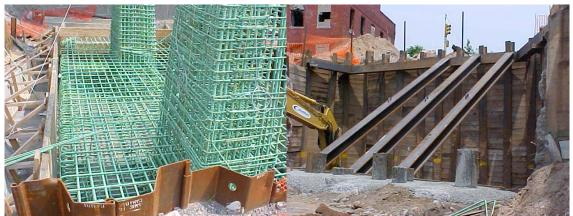
Installation of Footing and Column Reinforcement for the 2<sup>nd</sup> Avenue Bridge's Center Pier. Excavation Protection System at the North Abutment.
