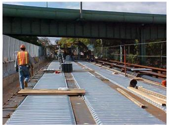
Installation of Stay-in-Place Deck Forms on the 2<sup>nd</sup> Avenue Bridge
