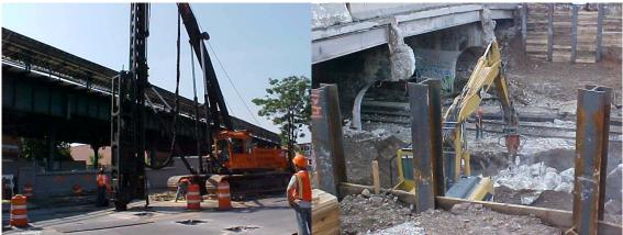
Installation of the Soldier Piles for the Excavation Protection System for the 14<sup>th</sup> Avenue Bridge. Excavation for the Abutment Footing.
