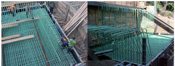
Installation of Abutment Footing and Stem Reinforcement for the 14th Avenue Bridge
