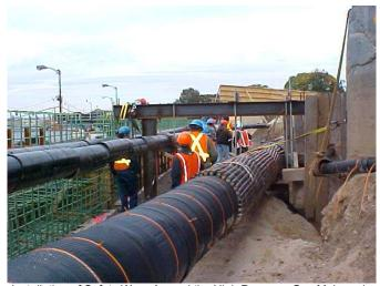
Installation of Safety Wrap Around the High Pressure Gas Main and the Con Edison Oil-o-Static Pipeline
