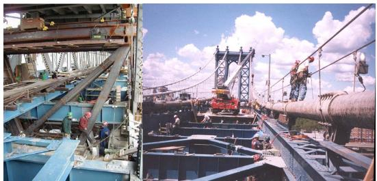
Contract #10 Temporary Truss Jacking Frame Used in the Work to Replace the Existing Truss Bearings.
