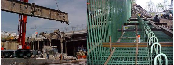
Demolition of the 2<sup>nd</sup> Avenue Bridge Superstructure. Abutment Footing and Stem Reinforcement.
