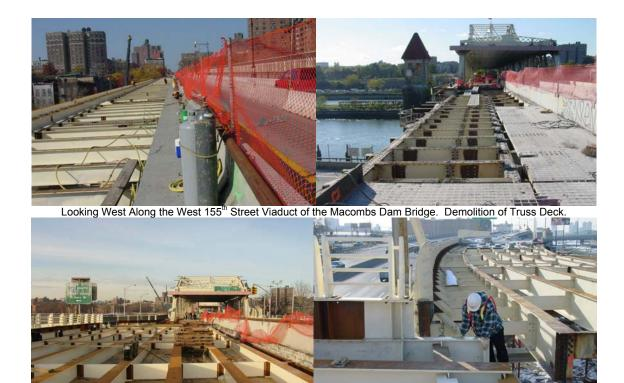
New Floor Beams in the East Approach of the Macombs Dam Bridge. Existing Steel Beams After Removal of Concrete on Ramp B.
