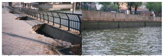
Severe Pavement Undermining and Collapse at 145<sup>th</sup> Street Due to Fill Loss Through Corroded Steel Sheet Piling. East River Bulkhead.
