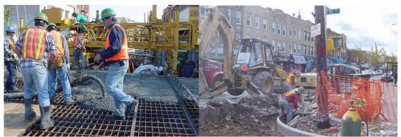
Placing Concrete for the 91<sup>st</sup> Place Bridge Grid Deck. Installation of New Sidewalk and Roadway at the Corner of Corona Boulevard and 91<sup>st</sup> Place.
