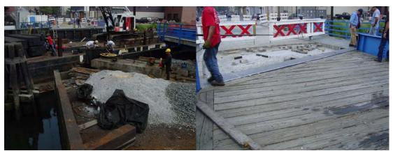
Gravel Pile to be Used as Backfill After Completion of Timber Replacement at the Carroll Street Bridge.
