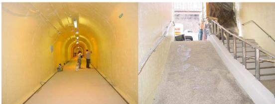
Applying the 2<sup>nd</sup> Skid Resistant Coating to the Western Half of the Tunnel Floor. Repaired Staircase With a Skid Resistant Coating on the Ramp and Landing. (Credit: Thomas Leung)
