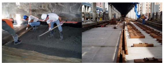
Placing the Waterproof Protection Layer on the Anchorage Roof Inside the North Track Envelope.
