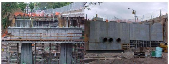
View of the Partially Completed Center Pier and South Abutment of the New 2<sup>nd</sup> Avenue Bridge. View of the New North Abutment Stem Wall.
