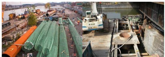
Third Avenue Bridge Rebar Cage Assembly and Staging Area.
