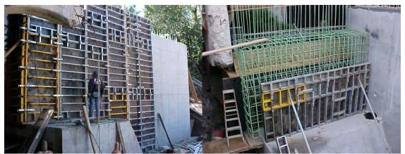
View of Reinforcement and Form Work Installation at the 14<sup>th</sup> Avenue Bridge Abutment
