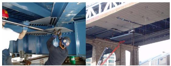
Torquing the Bolts for the Installation of the Upper Laterals for the Truss Stiffening System.
