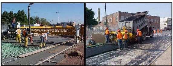
Placing Concrete for the New Grand Avenue Bridge Deck. Paving the Asphalt on the New Approach Slabs.
