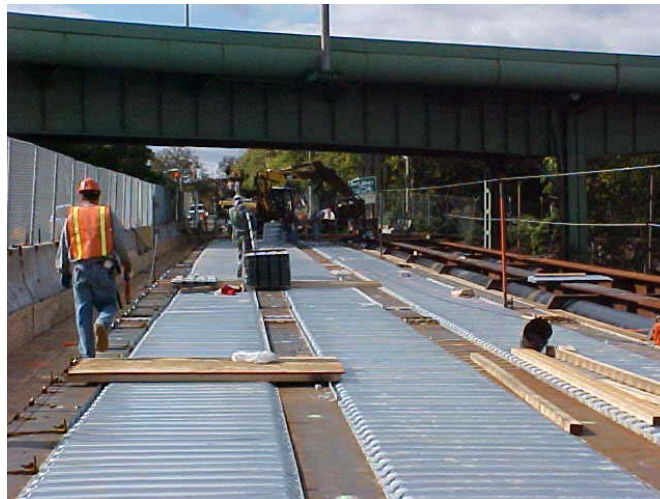
Installation of Stay-in-Place Deck Forms on the 2 nd Avenue Bridge
