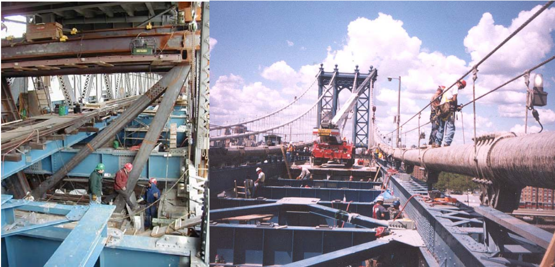
Contract #10 Temporary Truss Jacking Frame Used in the Work to Replace the Existing Truss Bearings. Replacement of Steel Stringers and Floorbeams on the North Upper Roadway Main Span.
