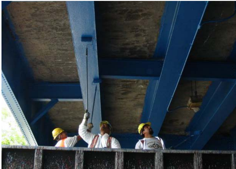
Bridge Painters Milan Radovic, Goncarlo Lima, and Samuel Martinez applying the Finishing Touches on the Beams of the Belt Parkway Bridge over Ocean Avenue. (Credit: Lisi de Bourbon)
