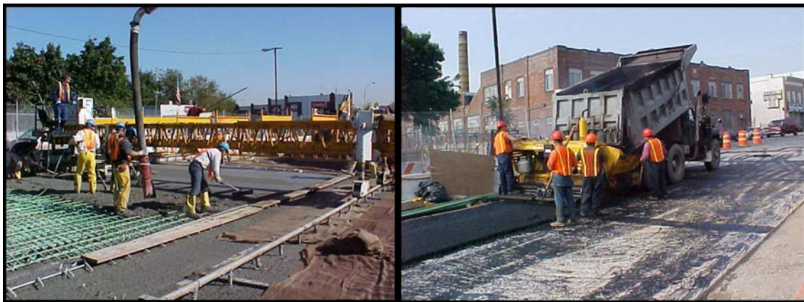
Placing Concrete for the New Grand Avenue Bridge Deck. Paving the Asphalt on the New Approach Slabs.
