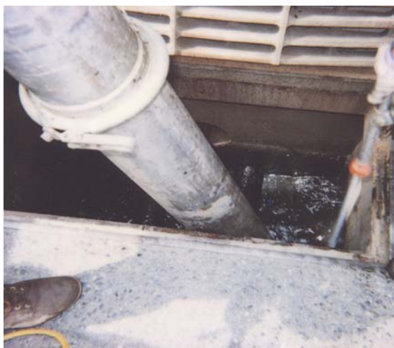
Cleaning Catch Basins on the Manhattan Bridge
