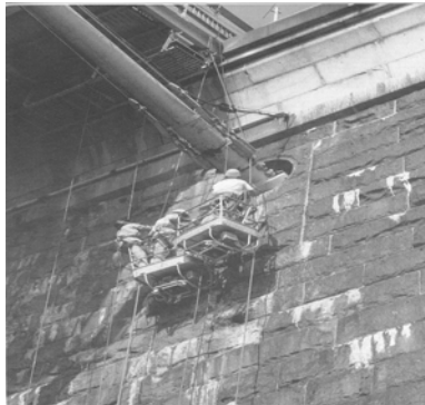
Consultants Inspecting the Splay Casting at Anchorage D of the Williamsburg Bridge, Where the Suspension Cables are Secured
