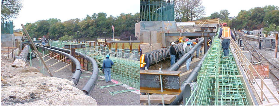
Installation of Reinforcement in the 7 th Avenue Bridge Abutment Stem and Backwall
