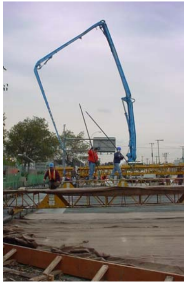
Placing Concrete for the Cross Bay Boulevard Grid Deck
