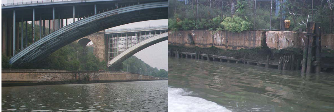
Bulkhead at Alexander Hamilton Bridge. Severe Erosion of the Concrete Seawall Allowing Loss of Fill at the MTA Rail Yard at 151 st Street.
