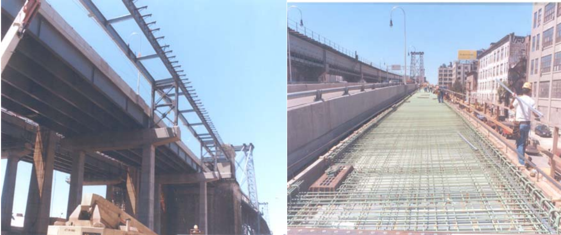
Contract #7 Bikeway Steel Erection & Rebar Installation
