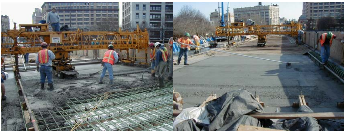
Placing and Finishing Concrete on the Grid Deck of the Brooklyn Elevated Structure.
