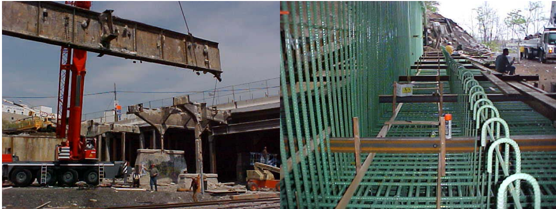
Demolition of the 2 nd Avenue Bridge Superstructure. Abutment Footing and Stem Reinforcement.
