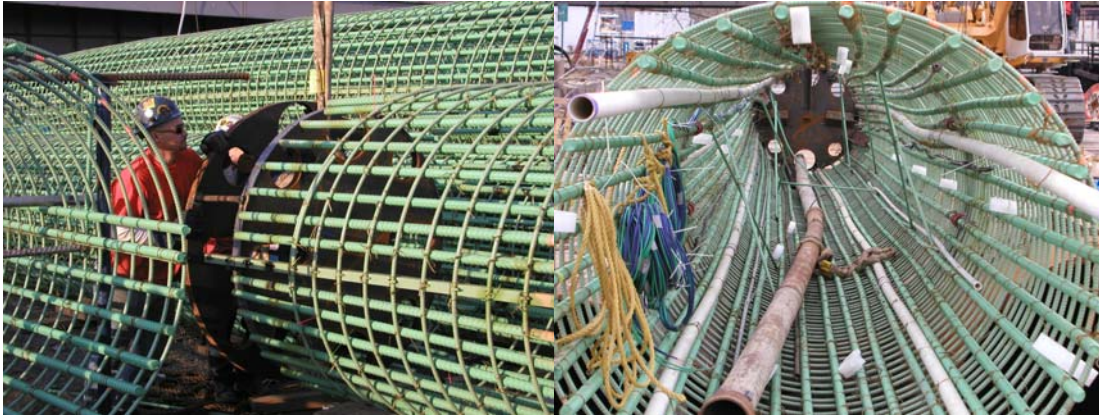
Osterberg Load Cell and Bearing Plate at Bottom of Reinforcing Cage. Instrumentation, Integrity Testing Tubes, And Concrete Tremie Pipe Within A Completed Reinforcement Cage.
