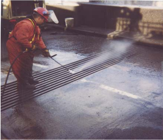
Expansion Joint Cleaning on the Manhattan Bridge
