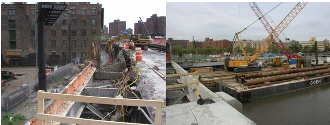
Third Avenue Bridge Stairway Demolition. Working on the River to Construct a Temporary Platform.
