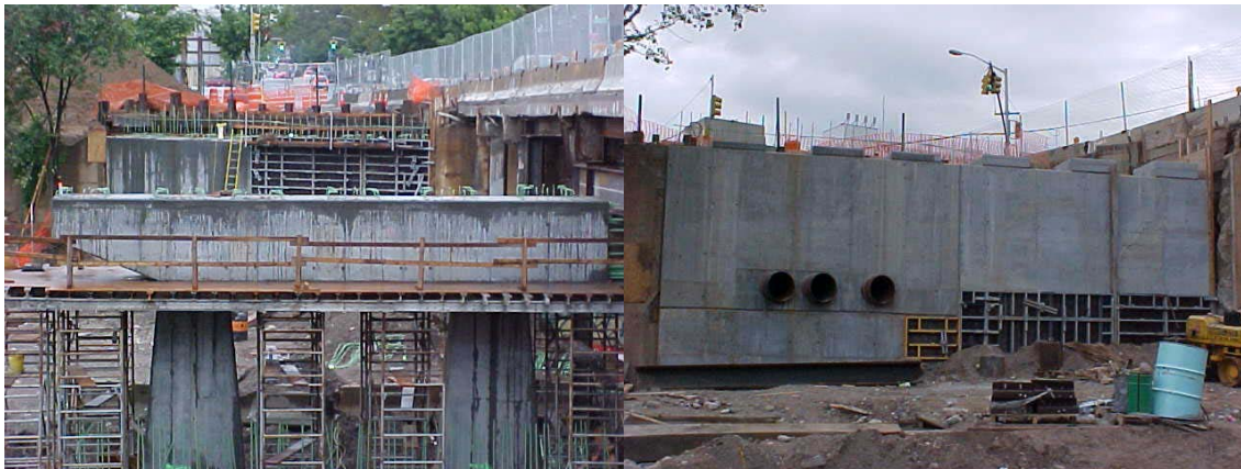
View of the Partially Completed Center Pier and South Abutment of the New 2 nd Avenue Bridge. View of the New North Abutment Stem Wall.
