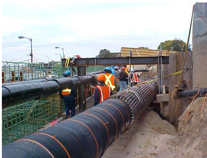
Installation of Safety Wrap Around the High Pressure Gas Main and the Con Edison Oil-o-Static Pipeline
