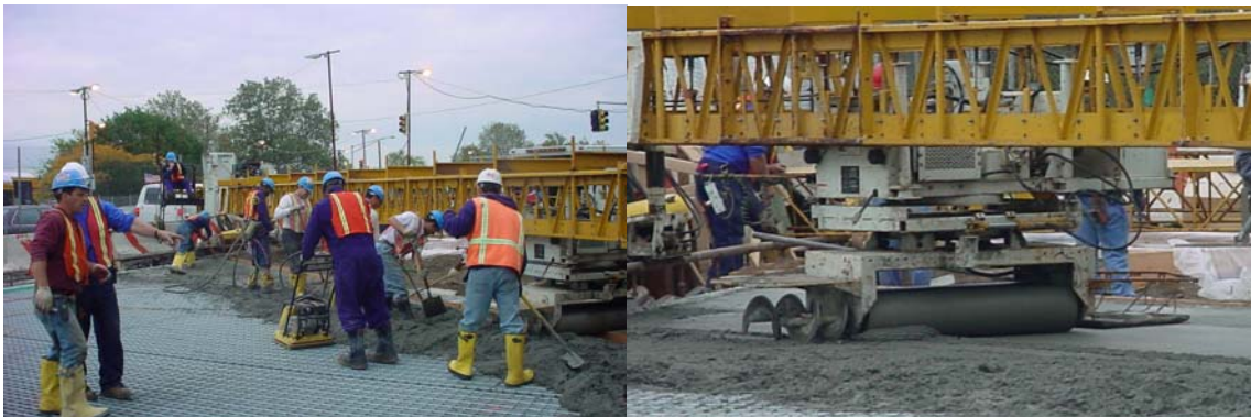
Placing Concrete for the Grid Deck of the Cross Bay Boulevard Bridge
