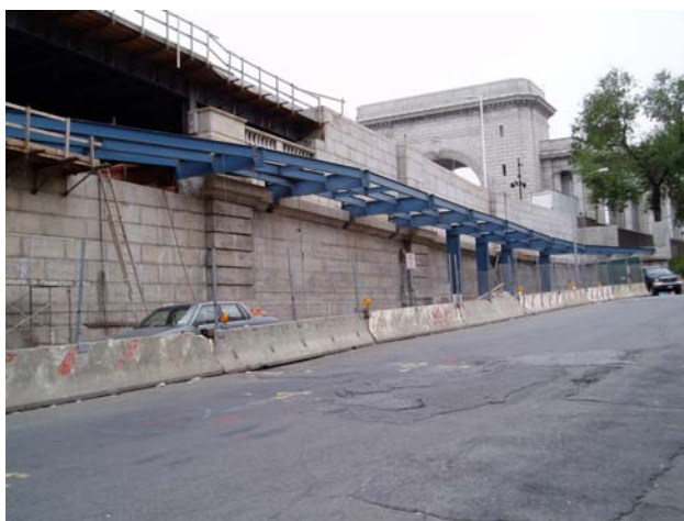
Construction of the New Bikeway Approach Ramp in Manhattan
