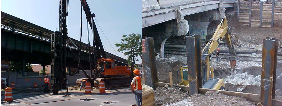
Installation of the Soldier Piles for the Excavation Protection System for the 14 th Avenue Bridge. Excavation for the Abutment Footing.
