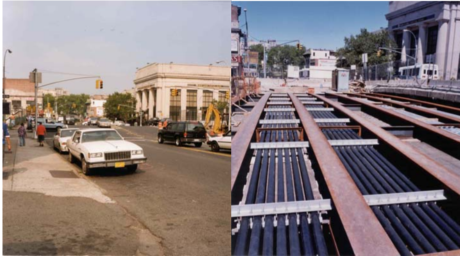
East Tremont Avenue Bridge Before Reconstruction. New ECS Conduits.
