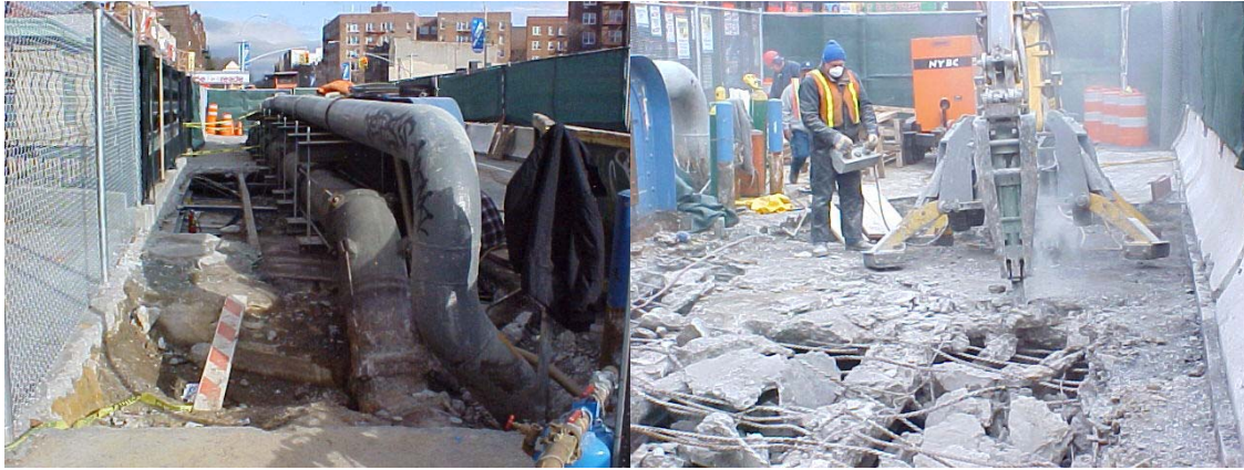
Demolition of the Cortelyou Road Bridge North Sidewalk. Demolition of the North Roadway.
