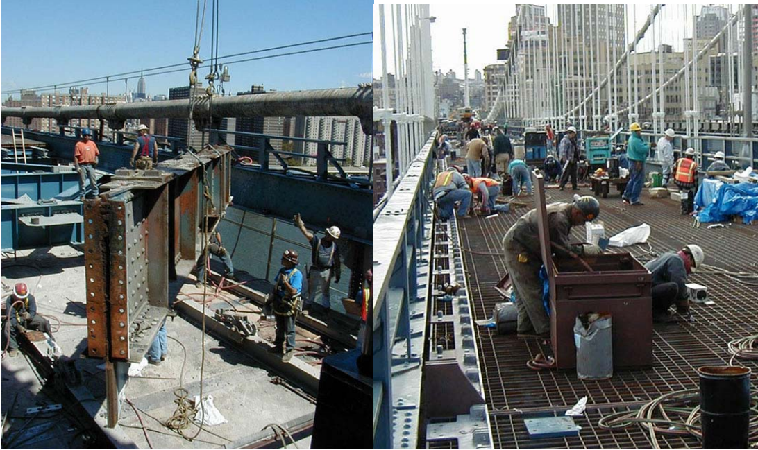
Contract #10 Removing an Existing North Upper Roadway Floorbeam on the Main Span of the Bridge. Installing the New Grid Deck for the North Upper Roadway on the Brooklyn Side Span.
