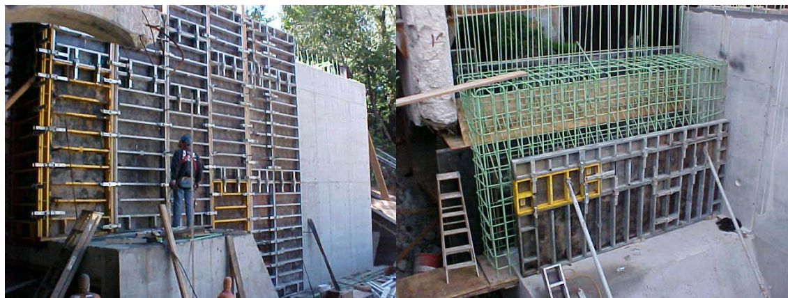
View of Reinforcement and Form Work Installation at the 14 th Avenue Bridge Abutment
