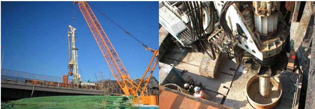
Drill Rig Installing the Third Avenue Bridge Manhattan Rest Pier Shaft from the Existing Bridge Deck. The Rebar Assembly and Staging Area are in the Foreground. Drill Rig Excavating the Drilled Shaft at the Center Pivot Pier.
