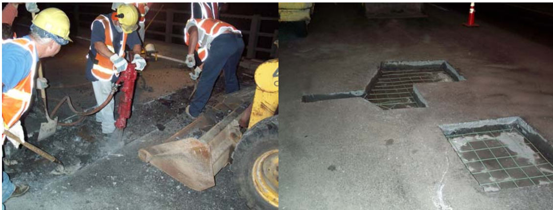
Concrete Deck Pothole Repairs Along the Westbound BQE Over Furman Street – Break-Out. Cutout Ready for Concrete. (Credit: Joseph Saverino)
