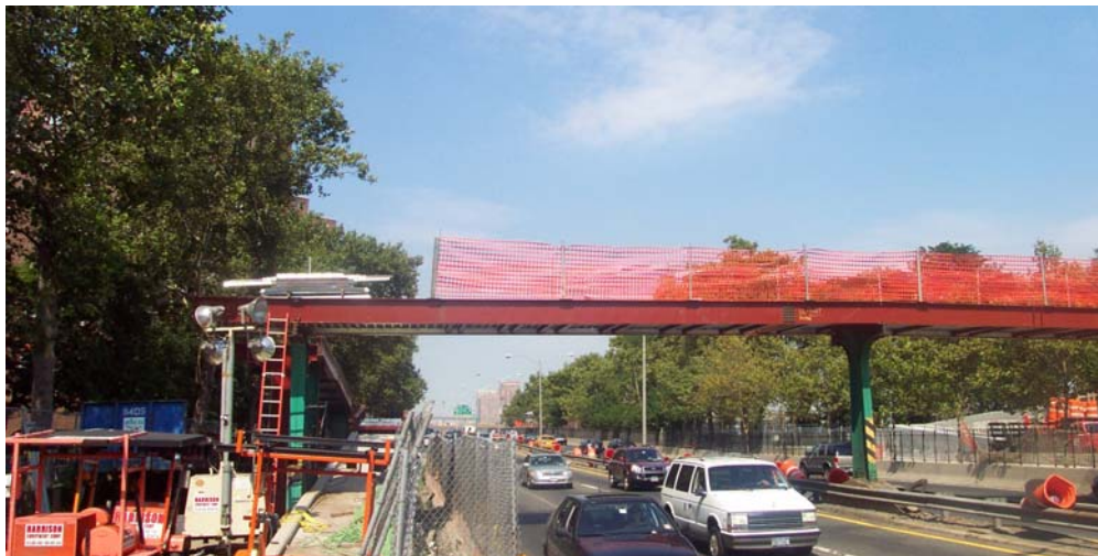
Erection of Structural Steel at the East 10 th Street Bridge (Credit: Bojidar Yaney)
