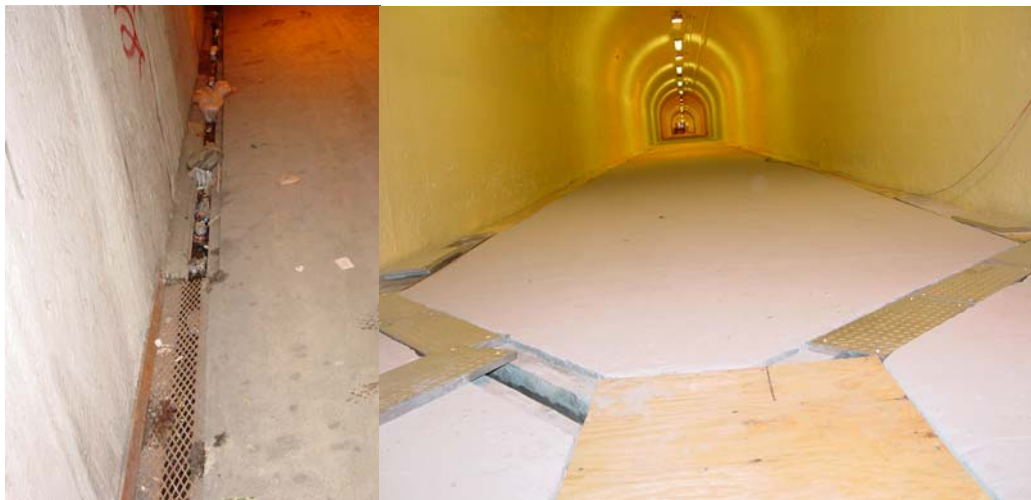
Old Drainage Grate Covers in the Eastern Half of the 191 st Street Tunnel. New Galvanized Grate Covers. (Credit: Thomas Leung)
