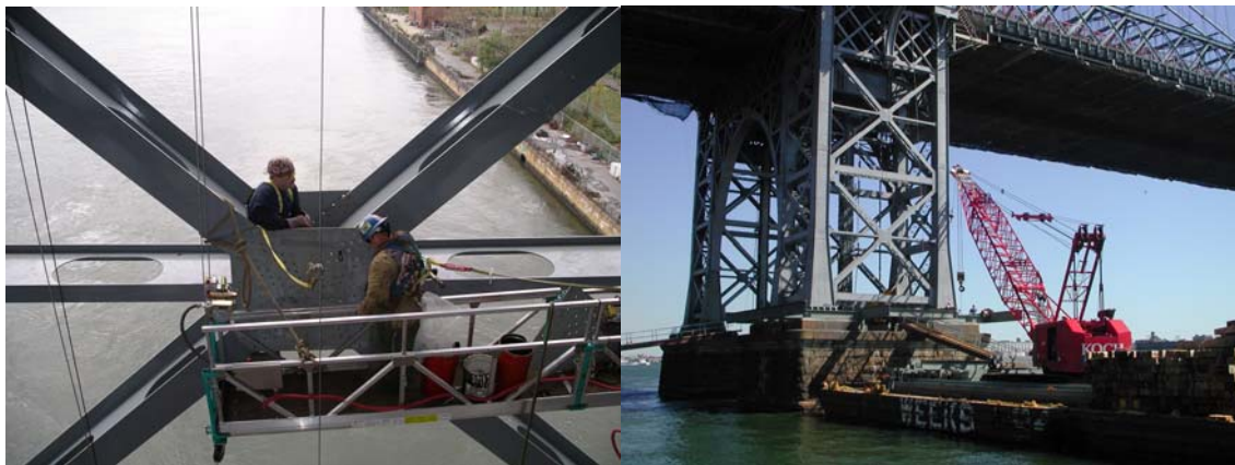
Contract #8 Manhattan Main Tower Member Replacement. Manhattan Main Tower South Pier Platform Erection.
