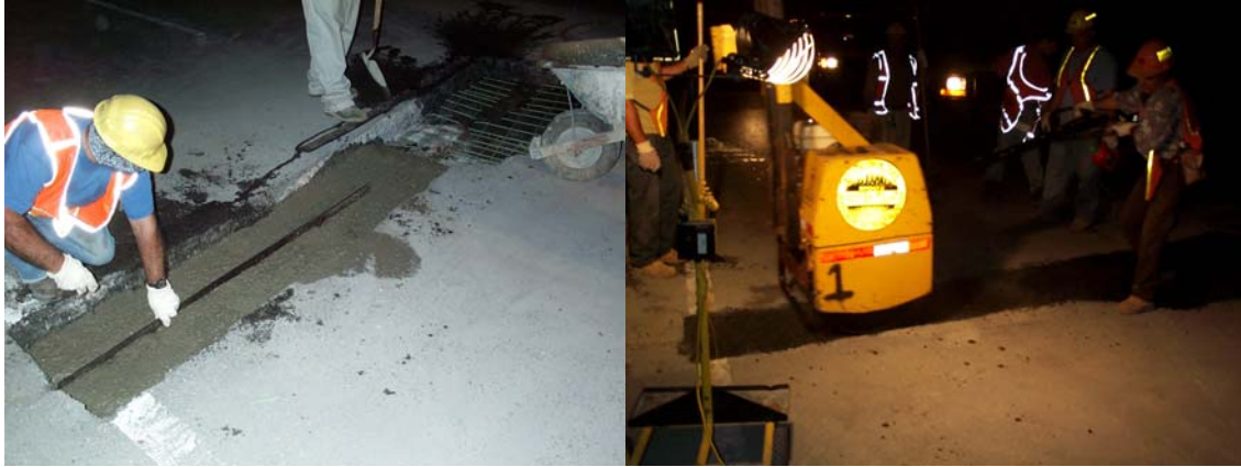
Pouring Concrete on the Westbound BQE Over Furman Street. Rolling and Tamping the Asphalt. (Credit: Joseph Saverino)
