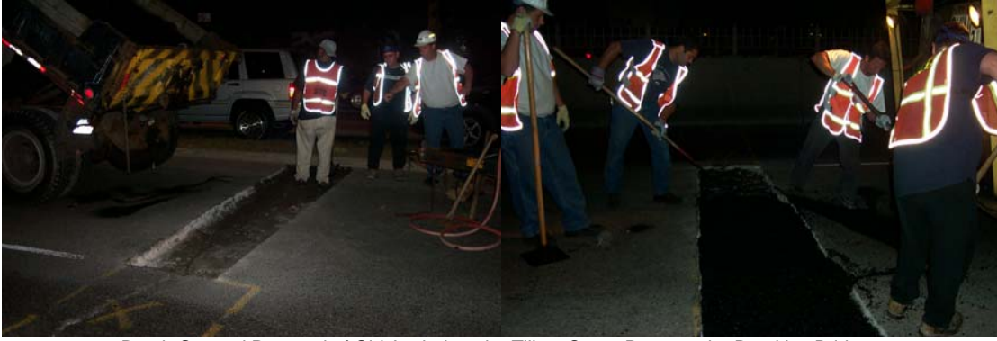
Break-Out and Removal of Old Asphalt at the Tillary Street Ramp to the Brooklyn Bridge (Credit: Anthony Napolitano)
