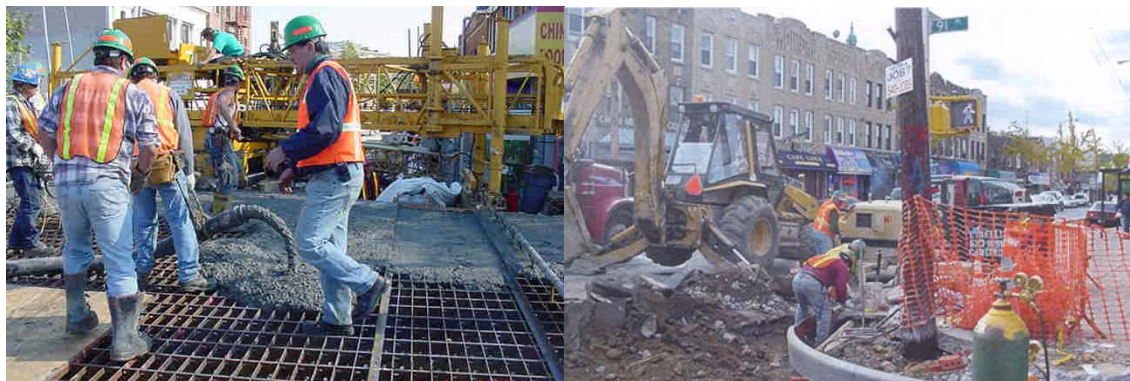
Placing Concrete for the 91 st Place Bridge Grid Deck. Installation of New Sidewalk and Roadway at the Corner of Corona Boulevard and 91 st Place.
