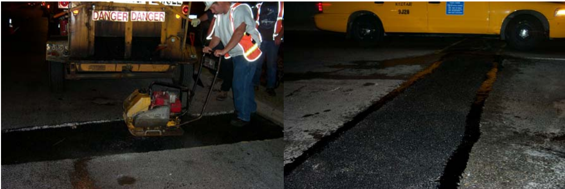
Compacting the Hot Asphalt Cement With a Portable Gasoline Powered Roller. Completed Asphalt Deck Repair at the Tillary Street Ramp. (Credit: Anthony Napolitano)
