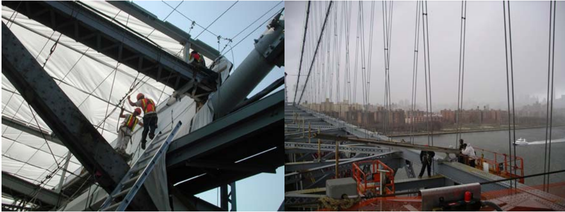
Contract #8 North Stiffening Truss Containment Erection and Removal
