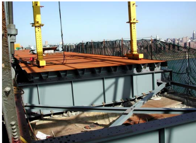
Contract #7 Installing An Orthotropic Deck Panel
