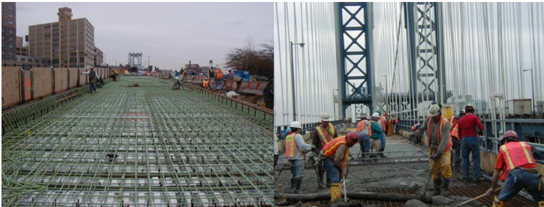
Preparing the Brooklyn Elevated Structure Grid Deck for Concrete Placement. Placing Concrete on the Manhattan Side Span Grid Deck of the North Upper Roadway.
