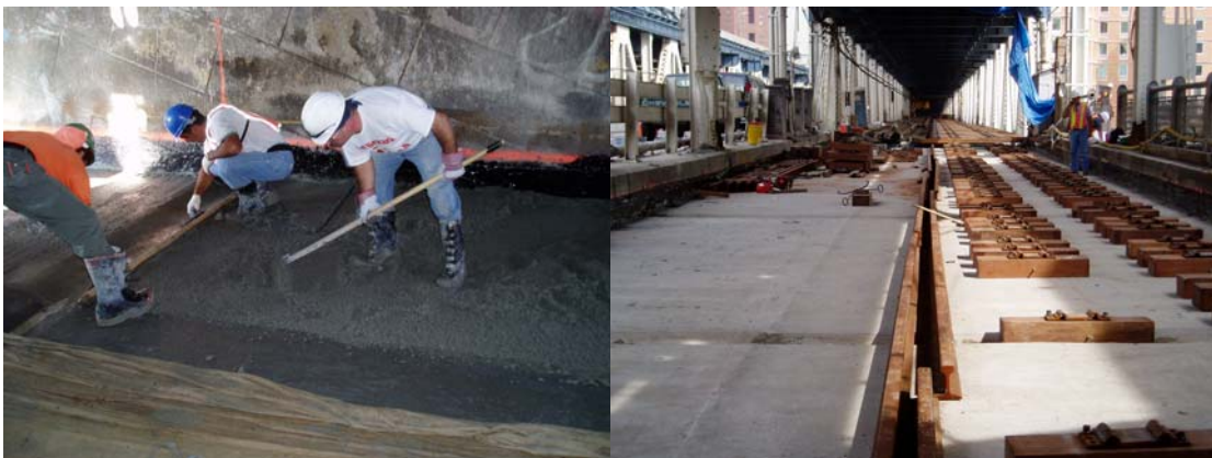
Placing the Waterproof Protection Layer on the Anchorage Roof Inside the North Track Envelope. Installation of New Ties for the North Subway Track.
