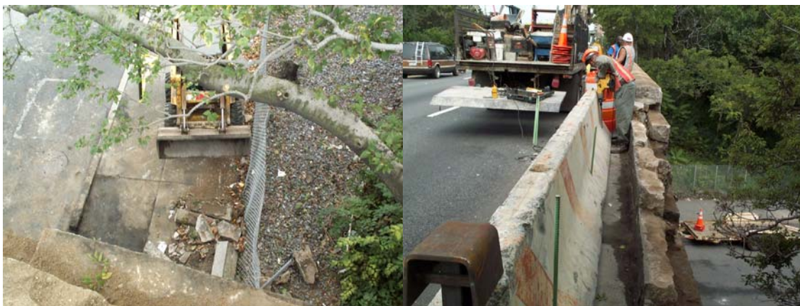
Clearing the Debris Below the Parapet. Drilling and Installing Pins Into the Jersey Barriers (Credit: Joseph Saverino)
