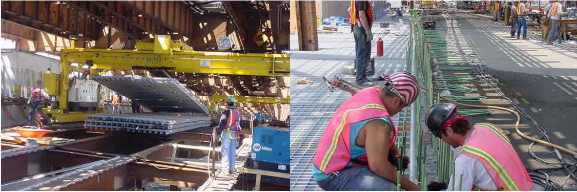
Queens Boulevard - Hoisting a Roadway Grating for Transport & Installing Electrical Conduits in a New Concrete Barrier
