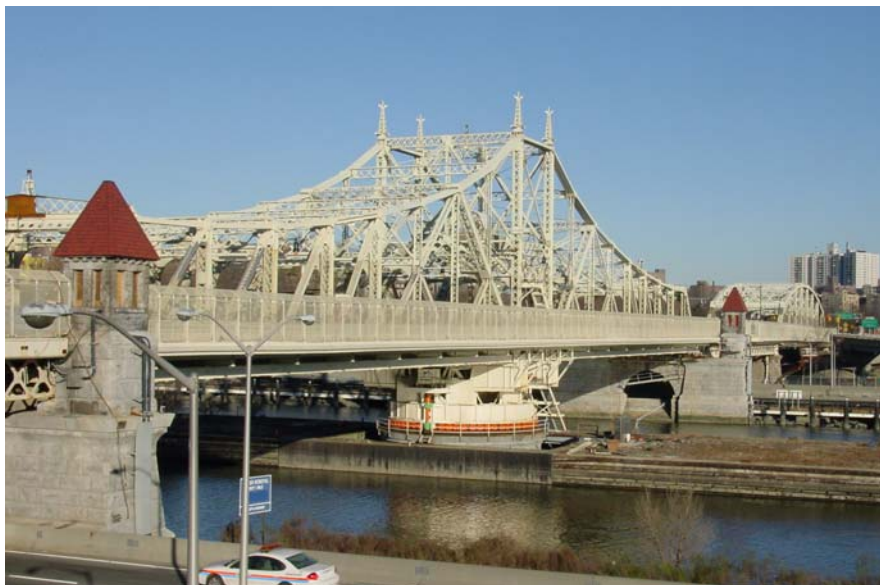
East View of Macombs Dam Bridge Swing Span and Camelback Truss (Credit: Hani Faouri)
