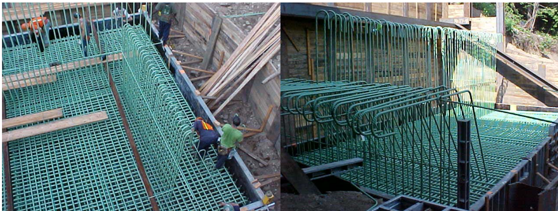
Installation of Abutment Footing and Stem Reinforcement for the 14 th Avenue Bridge
