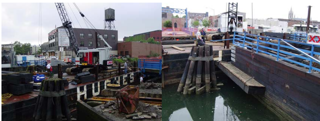
Work Barge Used During Carroll Street Bridge Repairs. Work Platform From Which the Timbers Were Replaced. (Credit: Thomas Leung)
