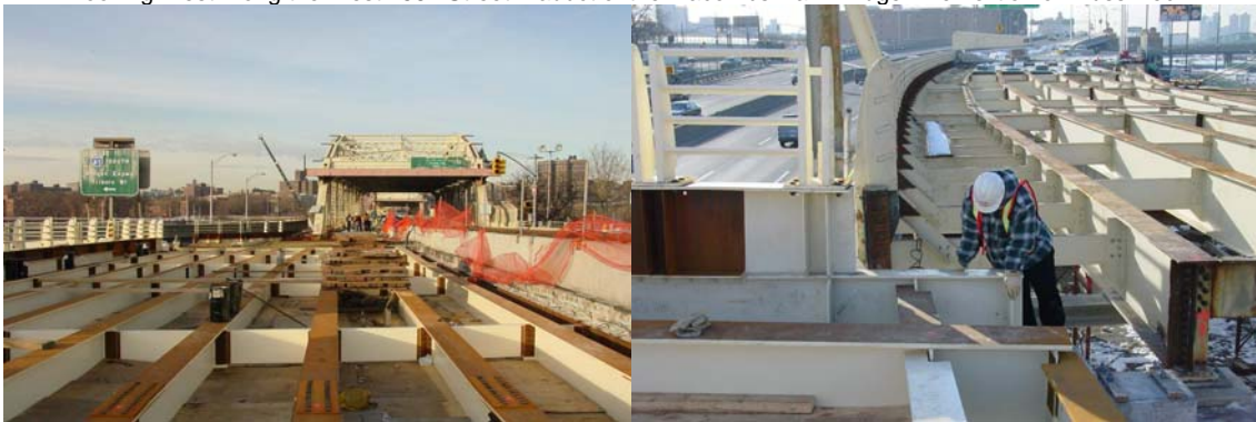
New Floor Beams in the East Approach of the Macombs Dam Bridge. Existing Steel Beams After Removal of Concrete on Ramp B.
