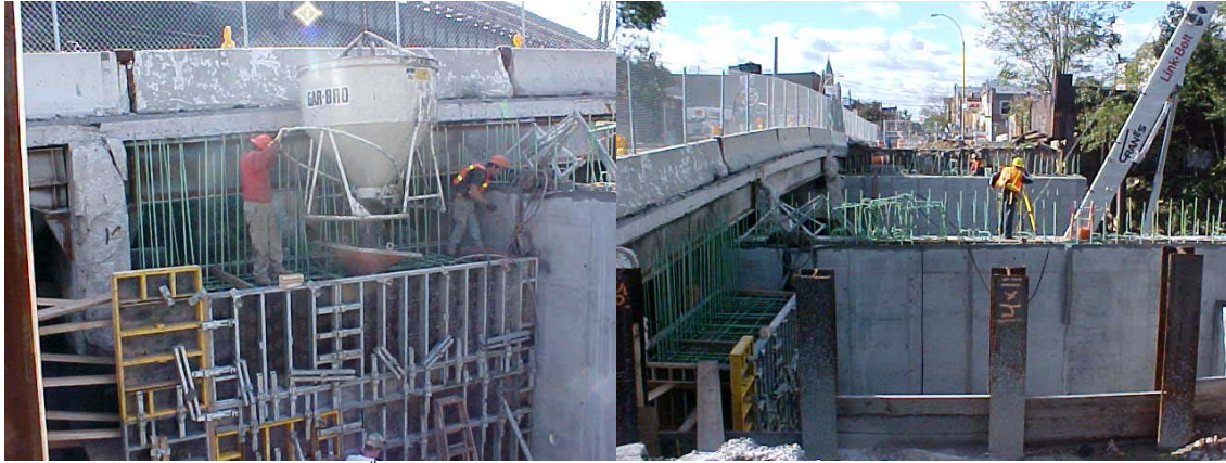
Concrete Pour at the 14 th Avenue Bridge Abutment. View of the Partially Completed Abutments.
