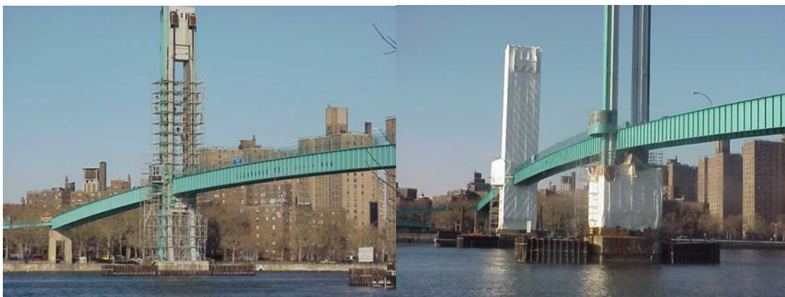
Tower Scaffolding and Containment at the Wards Island Pedestrian Bridge
