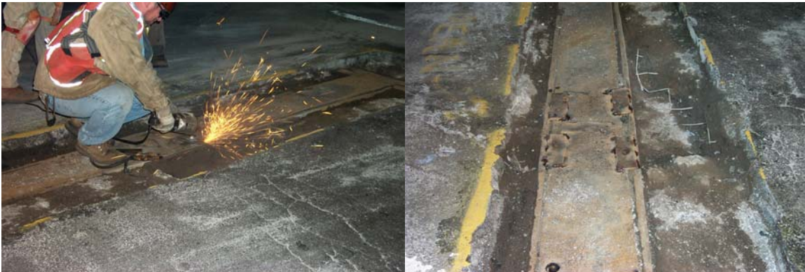
Repairing the Expansion Joint. (Credit: Anthony Napolitano)
