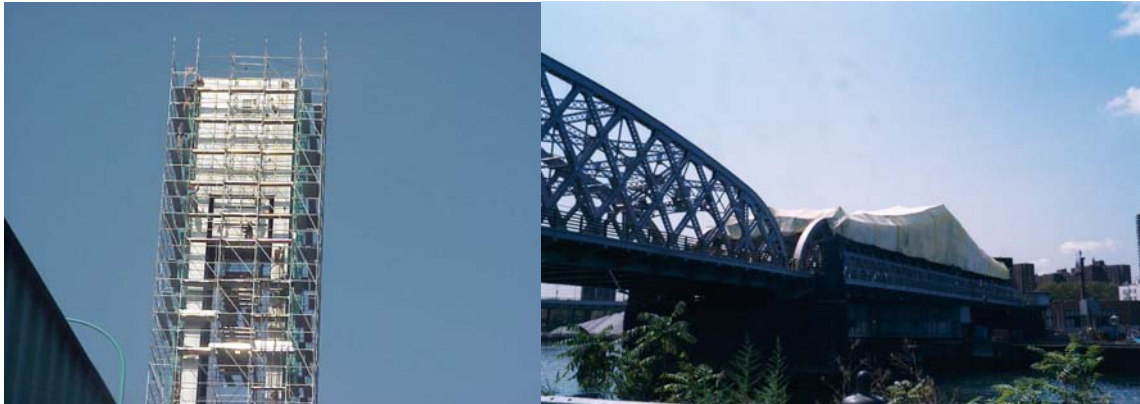
Wards Island Pedestrian Bridge Tower Scaffolding. Willis Avenue Bridge Containment.
