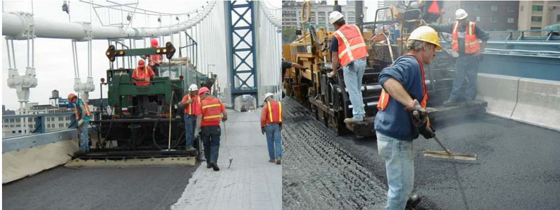
Placing the Microsurfacing Overlay on the Main Span. Placing the Asphalt Overlay on the Brooklyn Approach Span.
