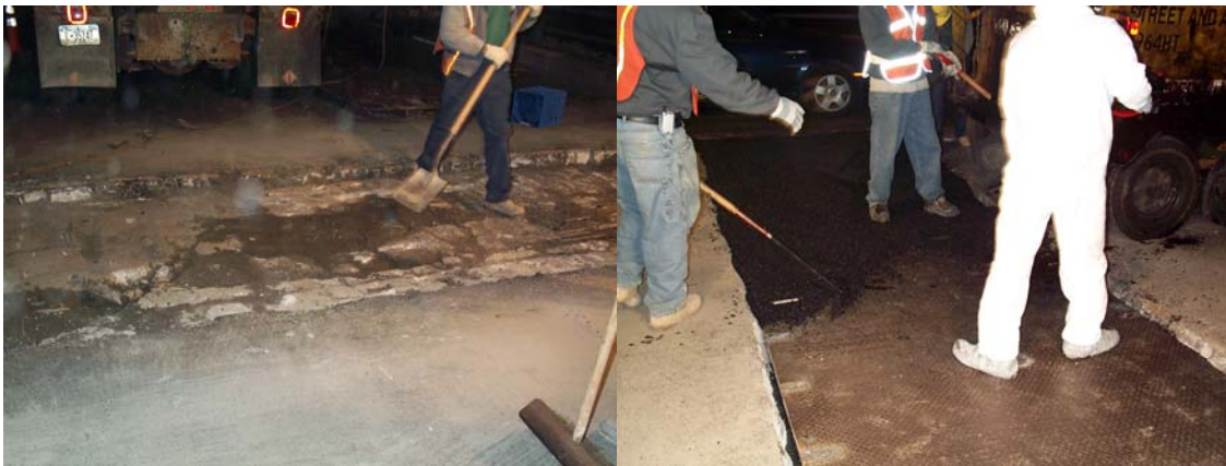
Side View of the Deteriorated Concrete to be Removed and Replaced. Placing Asphalt Over the Recessed Plates. (Credit: Joseph Saverino)
