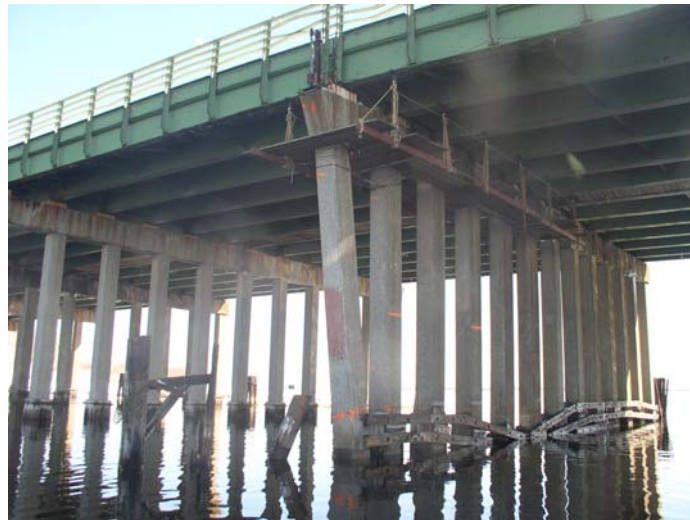
Broken Pier Column at the Belt Parkway Over Paerdegat Basin Bridge. (Credit: Bojidar Yanev)
