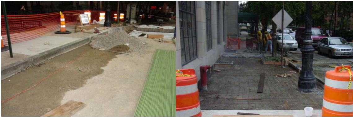
Concrete Base Course Repair and Sidewalk Repair at Tudor City Place Bridge (Credit: Nasir Khanzada)
