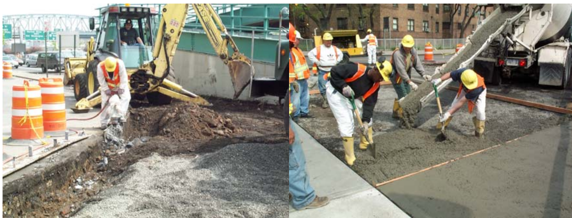
Highway Repairer Clifton Gravesande and Motor Grader Operator Robert Lovdhal Excavating With Pneumatic Hammer and Backhoe. Pouring Concrete for Sidewalk Replacement. (Credit: Joseph Saverino)
