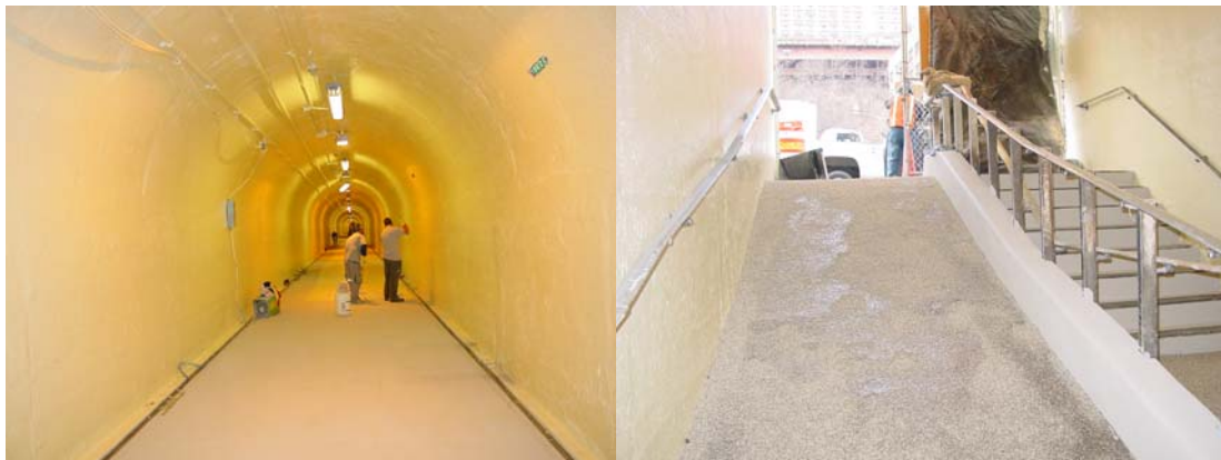
Applying the 2 nd Skid Resistant Coating to the Western Half of the Tunnel Floor. Repaired Staircase With a Skid Resistant Coating on the Ramp and Landing. (Credit: Thomas Leung)
