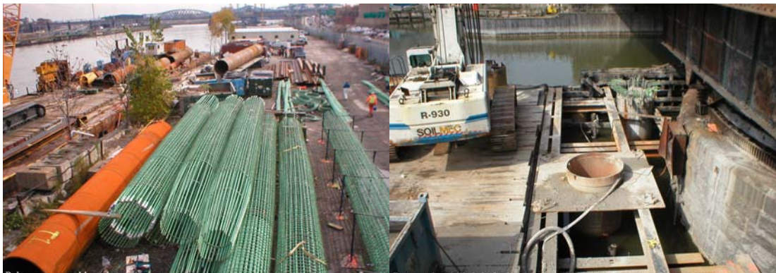
Third Avenue Bridge Rebar Cage Assembly and Staging Area. Constructing Drilled Shafts for the New Center Pivot Pier Foundation Adjacent to the Existing Pivot Pier.
