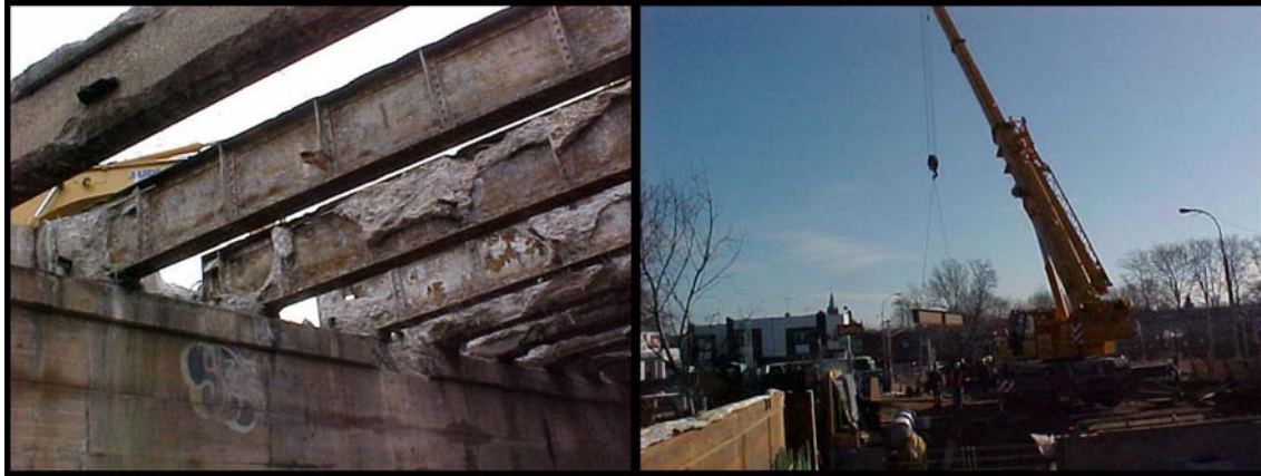
Demolition of the Grand Avenue Bridge. Erection of New Structural Steel.
