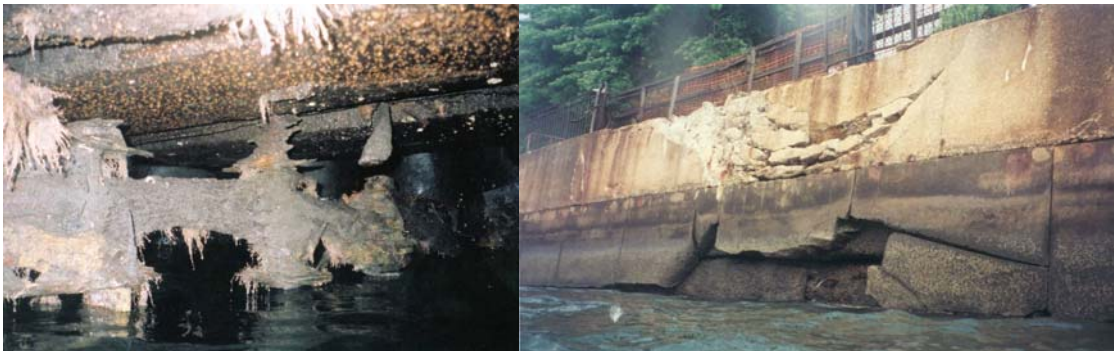
Deteriorated Pile Caps Under the Relieving Platform Adjacent to Pier 36. Severe Impact Damage to the Concrete Seawall and Stone Facing at the Foot of Cherry Street.
