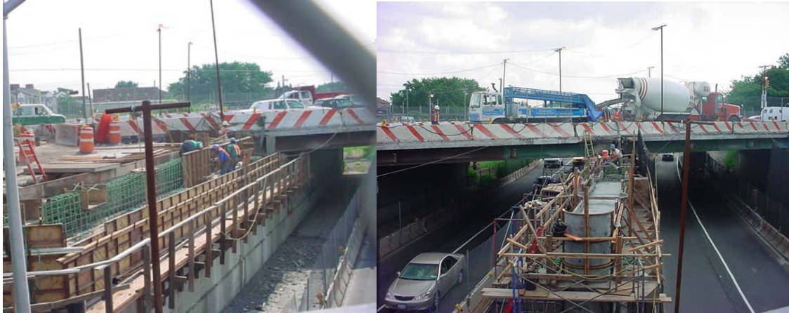
Construction of North Abutment Wall of the Cross Bay Boulevard Bridge. Placing Concrete for the Pier Cap.
