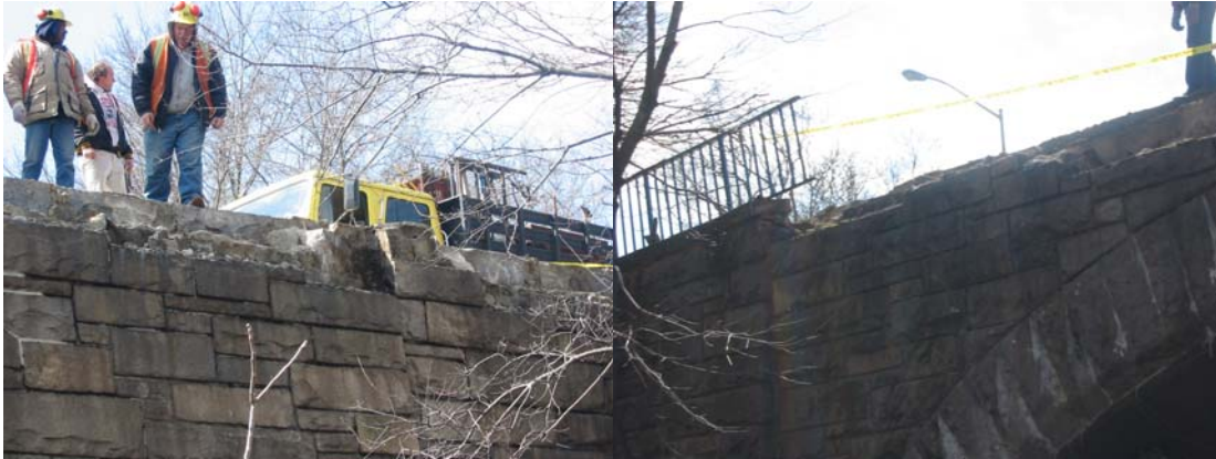
A Multi-Vehicle Accident Resulted in Damage to the Stone Cladding and About 200 Feet of Bridge Rail. (Credit: Wen Liao)
