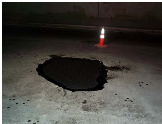
Closeup of Part of the Completed Concrete Deck Repair on the BQE. (Credit: Joseph Saverino)
