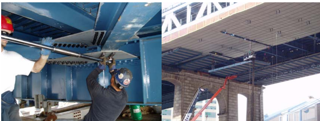
Torquing the Bolts for the Installation of the Upper Laterals for the Truss Stiffening System. Installation of a Permanent Maintenance Platform Under the Bridge on the Brooklyn Approach Span.
