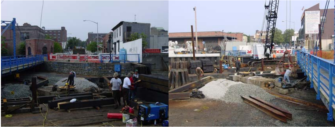
Cutting 12x12 Timbers On the Barge to Match the Wall. Clam Bucket Used for the Backfilling Operation at the Carroll Street Bridge. (Credit: Thomas Leung)
