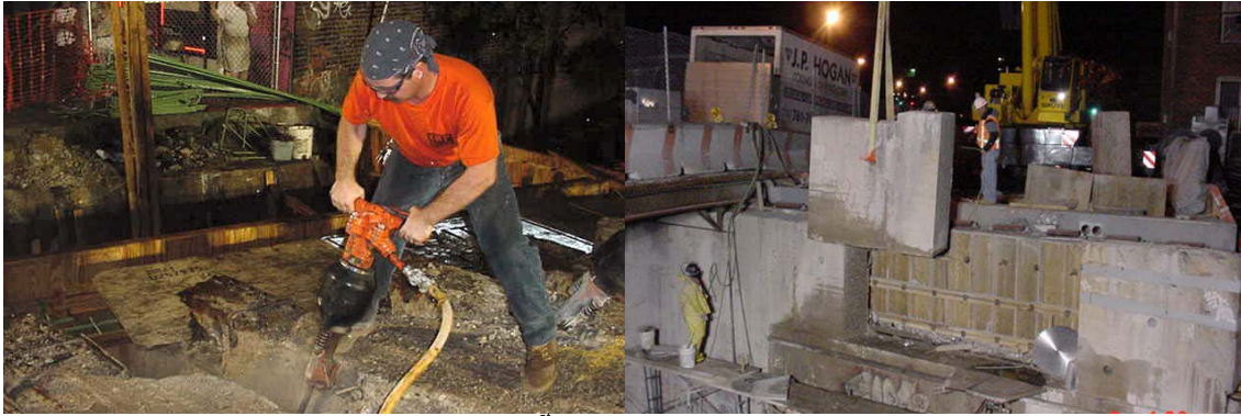
Exposing the Old Steel Stringer Ends on the 91 st Place Bridge. Removing the Central Pier by Saw Cutting the Concrete in Two Directions – Each Piece Weighed 9 Tons.
