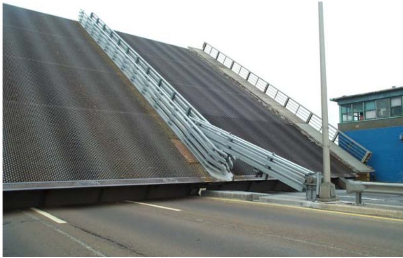
New Median Barrier of the Mill Basin Bridge (Credit: Vera Ovetskaya)
