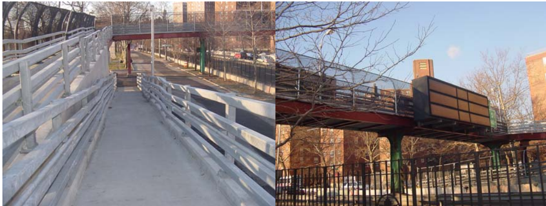
East Approach Lower Ramp of East 10 th Street Bridge. VMS Board Attached to North Fascia.
