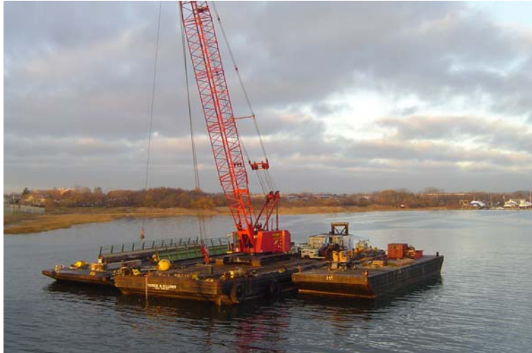
Barge and Crane Utilized in Paerdegat Avenue Bridge Repairs (Credit: Mansoor Khan)
