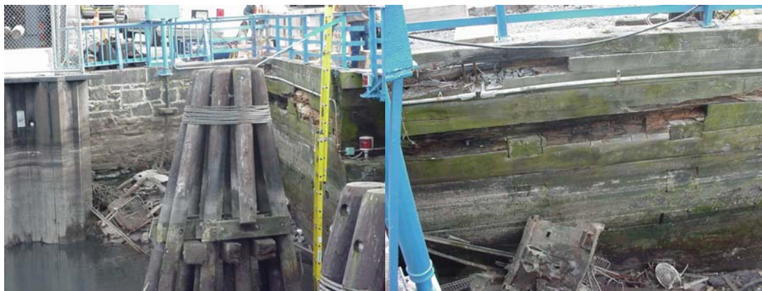
Carroll Street Bridge Before Repairs – Deteriorated Timber Walls Need Replacement. (Credit: Thomas Leung)
