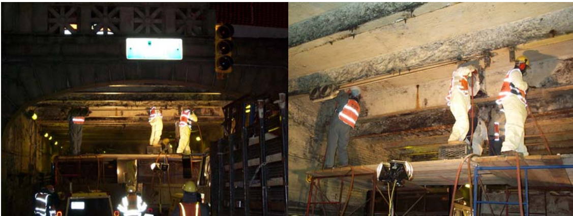
Masonry Crew Removing Concrete Encasement From a Steel Beam Inside the Park Avenue Tunnel (Credit: Joseph Saverino)
