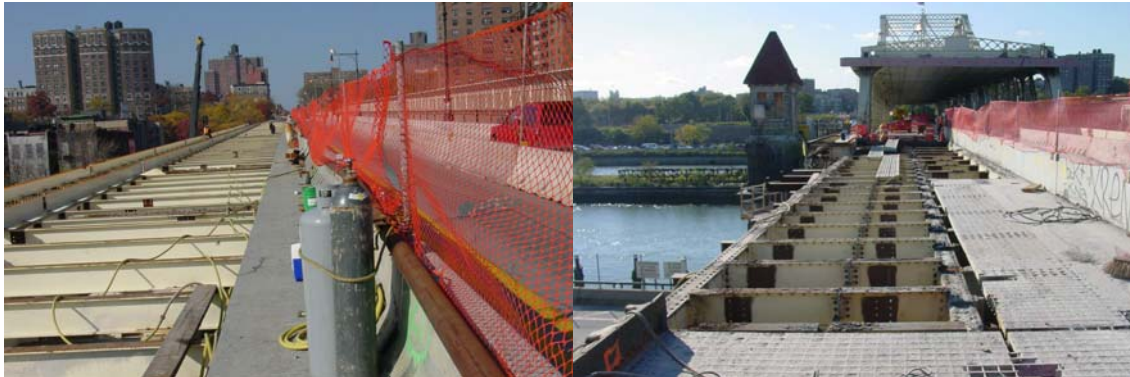
Looking West Along the West 155 th Street Viaduct of the Macombs Dam Bridge. Demolition of Truss Deck.
