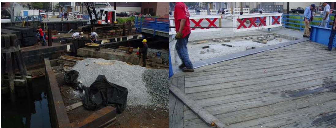
Gravel Pile to be Used as Backfill After Completion of Timber Replacement at the Carroll Street Bridge. Restoring the Paving Blocks in the Roadway. (Credit: Thomas Leung)
