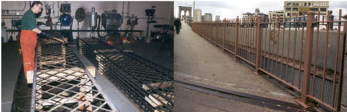
Painting the Replicated Railing. New Promenade Railing (Credit: Peter Basich)
