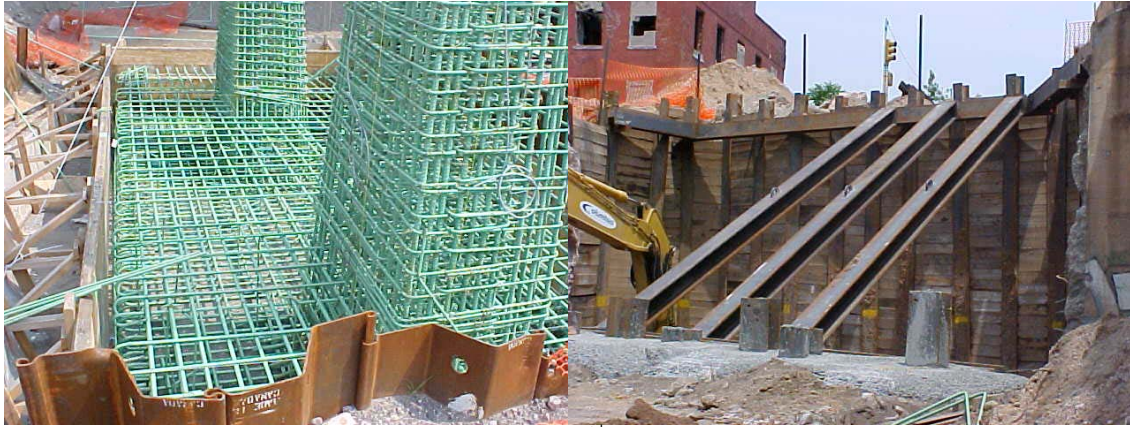
Installation of Footing and Column Reinforcement for the 2 nd Avenue Bridge's Center Pier. Excavation Protection System at the North Abutment.
