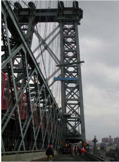
Contract #8 Manhattan Main Tower Temporary Platform Erection
