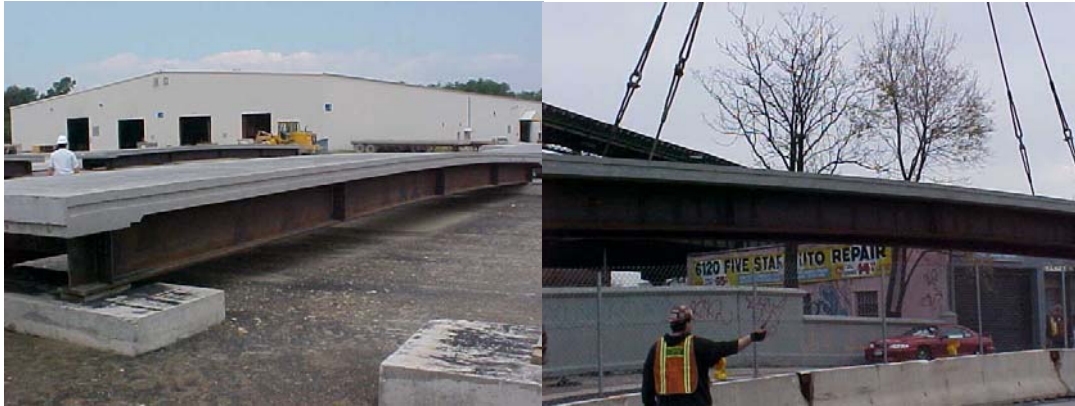
Precast Deck Panel in the Fabricator's Yard (Credit: Boowong Kim) Lowering the Panel Into Place.
