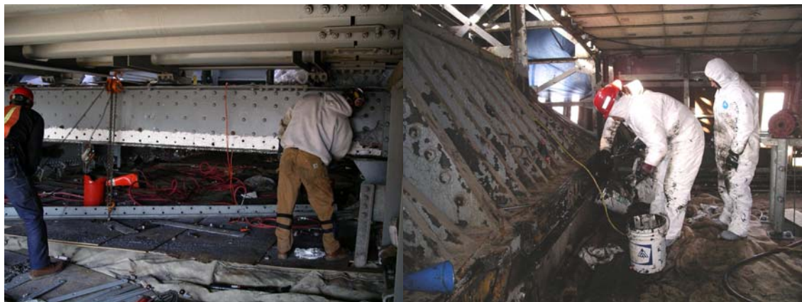
Contract #8 South Truss Bottom Chord Rehabilitation. .Degreasing the Brooklyn Main Tower Saddle Bearing.
