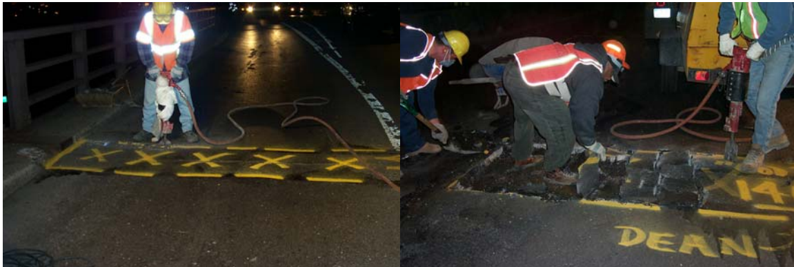
Breaking Out the Area With Jackhammers. (Credit: Anthony Napolitano)
