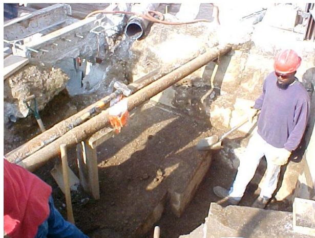
Excavation Behind the Abutments of the Cortelyou Road Bridge
