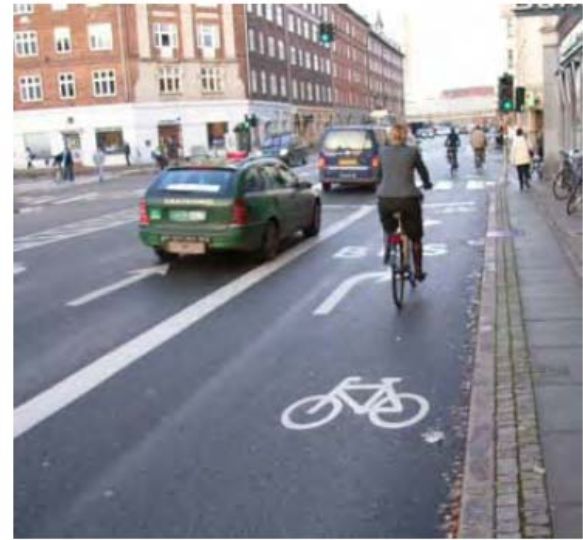
Figure 2. Photos of a shortened cycle track extended into a narrow cycle lane (left), an advanced cycle track with a blue cycle crossing and a pre-green light for cyclists (middle), a shortened cycle track extended into a right turn-lane (right).
