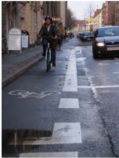
Figure 2. Photos of a shortened cycle track extended into a narrow cycle lane (left), an advanced cycle track with a blue cycle crossing and a pre-green light for cyclists (middle), a shortened cycle track extended into a right turn-lane (right).
