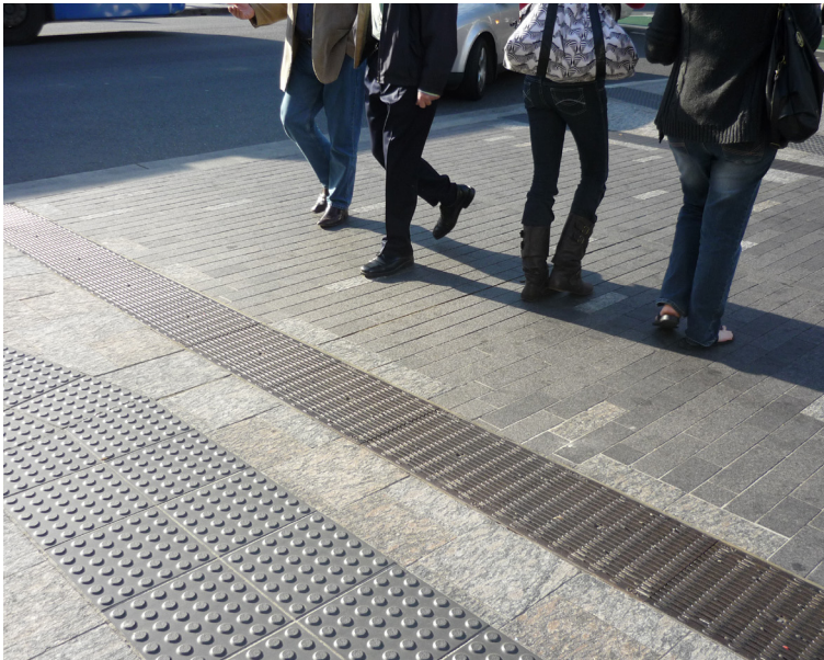
Detectable warnings at Albert Street, Brisbane, AU (source: Arup)
