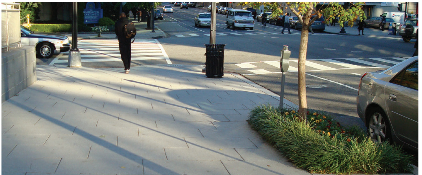
Scored Concrete, Washington DC (source: NYCDOT)
