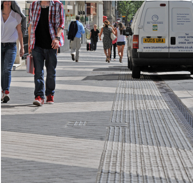
Tactile warning strips at Exhibition Road, London (source: Arup)
