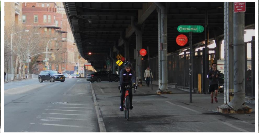
Greenway between Rutgers & Montgomery Sts lacks separation from vehicular traffic
