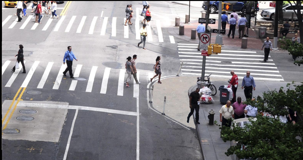
Example of painted curb extension:
