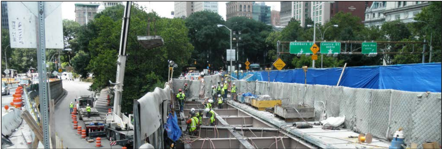
Demolition of roadway in preparation for placement of Pre-cast Grid-deck panels on Park Row Bridge Structure in Manhattan
