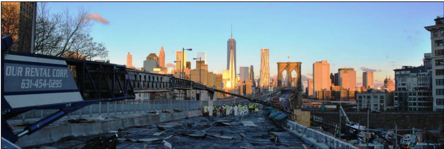
Full replacement of stringers and floor beams on York Street Bridge Structure in Brooklyn
