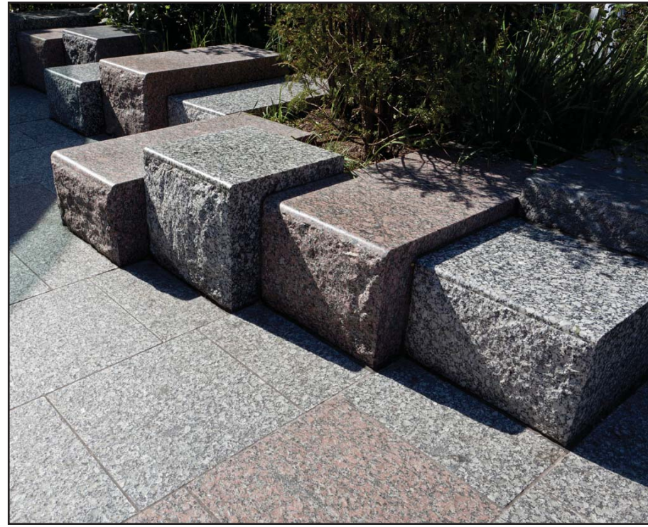
Item A. Stone Block Seating used at Edges of Planting Areas
