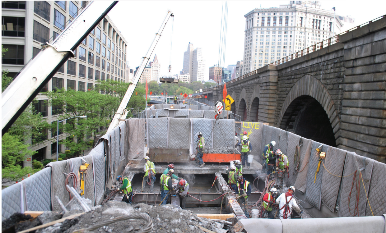
Two crews work along Frankfort St in April 2012. Cranes (on left) lift material in and out of walled enclosures of sound blankets.
