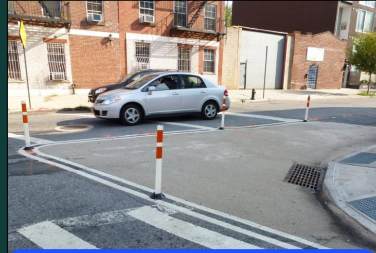
High Visibility Crosswalk and Flush Painted Sidewalk Extension: Washington Avenue, Brooklyn
