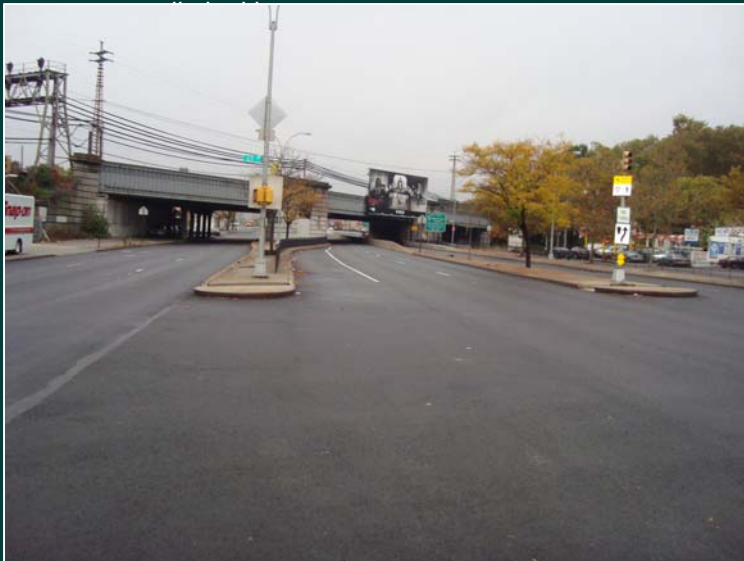
Queens Blvd & 69 th St, looking west
