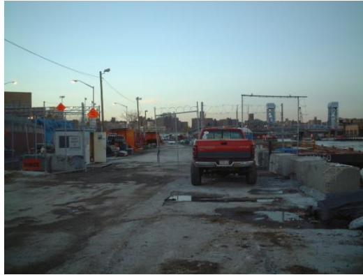
Construction staging area at waterfront
