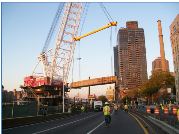
Old Bridge Span Removed on July 31
