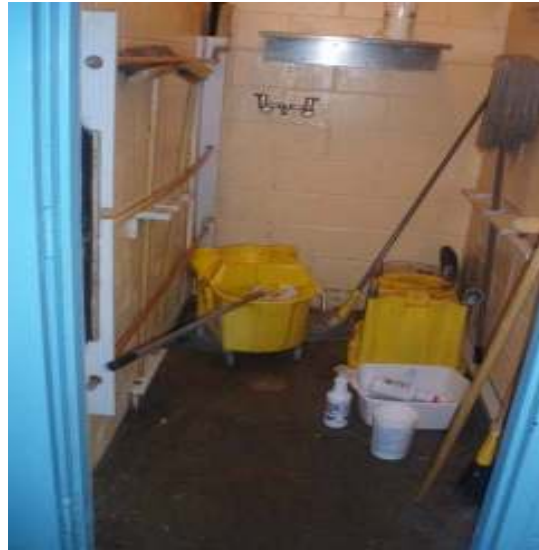
POORLY MAINTAINED JANITOR CLOSET
