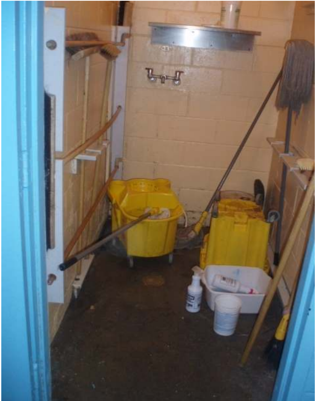
Poorly Maintained Janitor Closet
