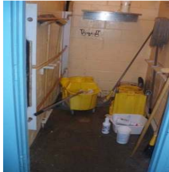
POORLY MAINTAINED JANITOR CLOSET
