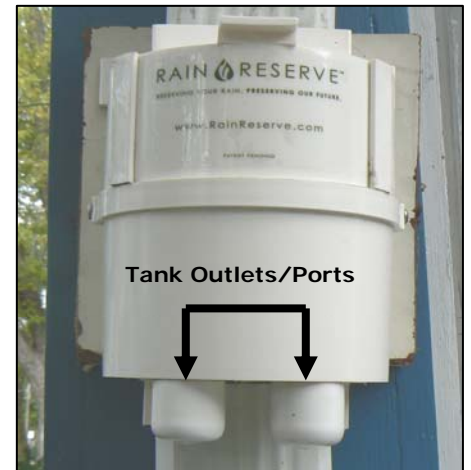
An Example of a Winterized Diverter
