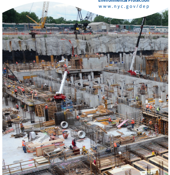
Construction of the Croton Water Filtration Plant under Mosholu Golf Course
