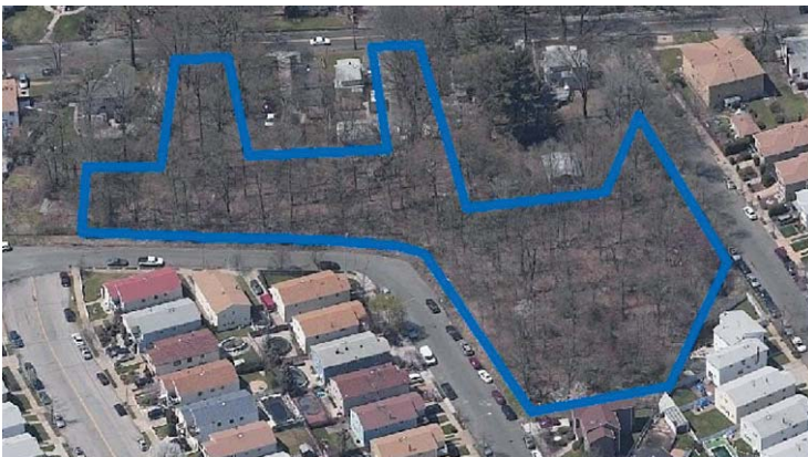
East side of Annadale Road 113 feet south of Laredo Avenue 3% in bed of street Vacant Lot Staten Island Parcel 48, page 45
