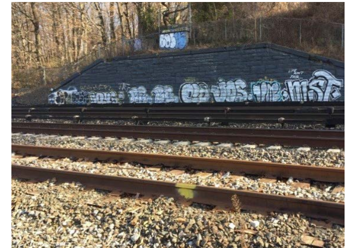
Photo A06: Looking northeast at surviving abutments of former pedestrian bridge near Riverdale Park / West 246th Street
