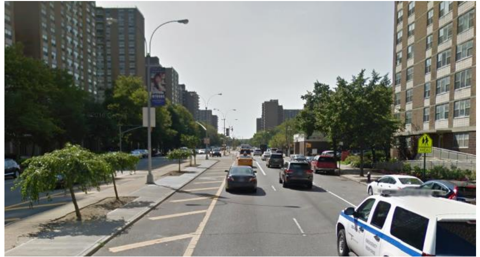
Pennsylvania Ave near Twin Pines Dr, looking south
