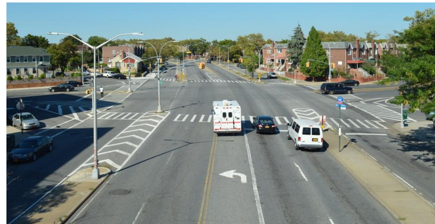
Kings Hwy at Ave K, looking northeast
