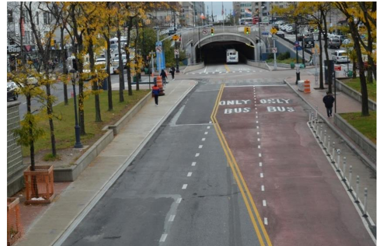
161 st Street Bus Only Tunnel (eastbound)
