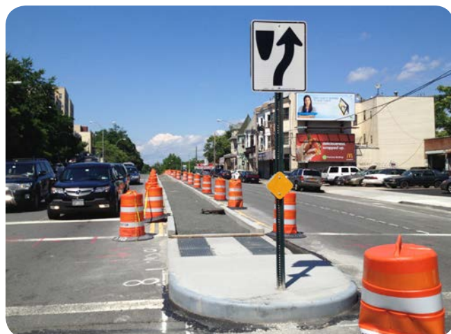
NYCDOT concrete crews built nine pedestrian refuges, two medians, and one sidewalk extension.
