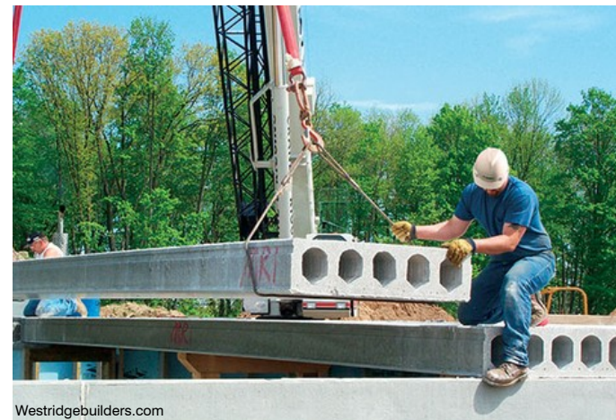
'Block and Plank' construction
