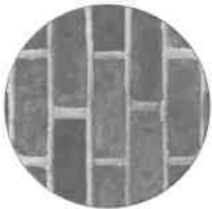
Original Red Brick After Paint Removal Brick Facade
