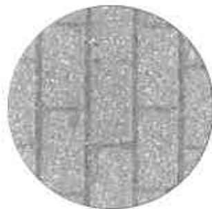
Existing Concrete Block Pavers for Reuse Pedestrian Path Near Spray Shower
