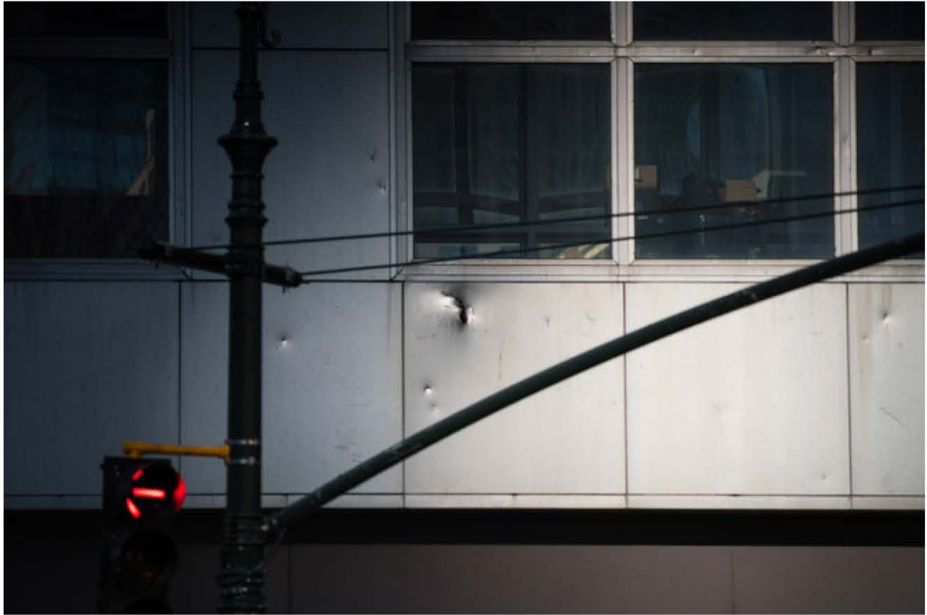
Dents on the north side of the pedestrian bridge. Credit Emon Hassan for The New York Times
