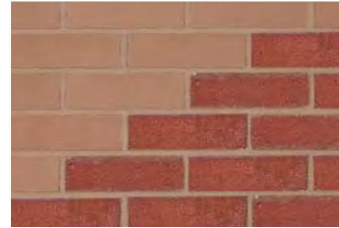
Brick - At Lot Line & Rear Wall
