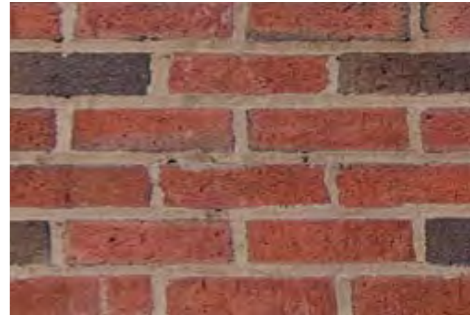
Brick - At Street Facade
