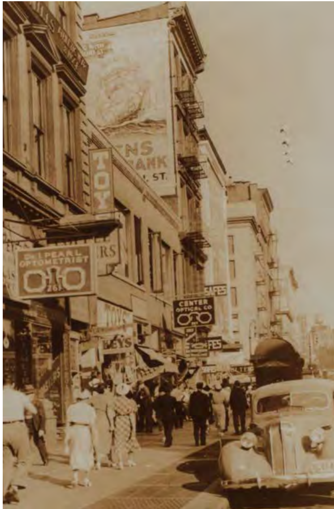
Canal Street near Broadway, 1937 (NYPL)
