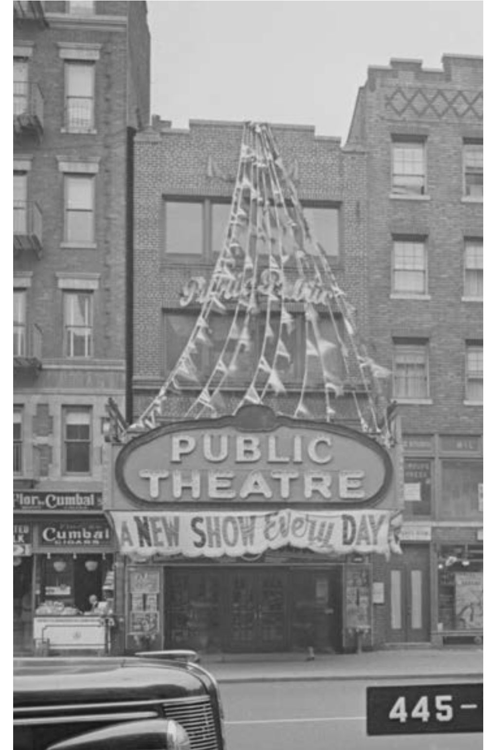
Public Theatre, 66 Second Avenue (H. Craig Severance, architect, David Oltarsh, consulting engineer, 1927)
