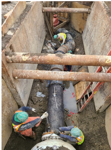
↑ The 20" distribution water main installation on Pelham Parkway North Service Road between White Plains Road & Boston Road.
