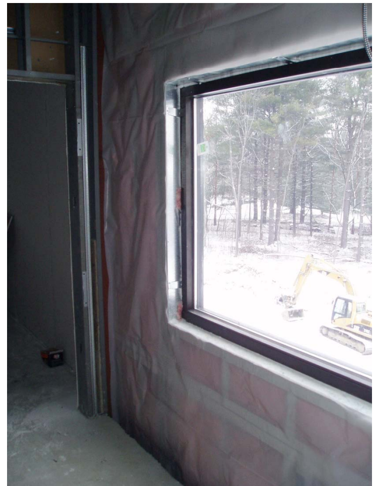
Class II Vapor Retarder Installed on Inside Face
