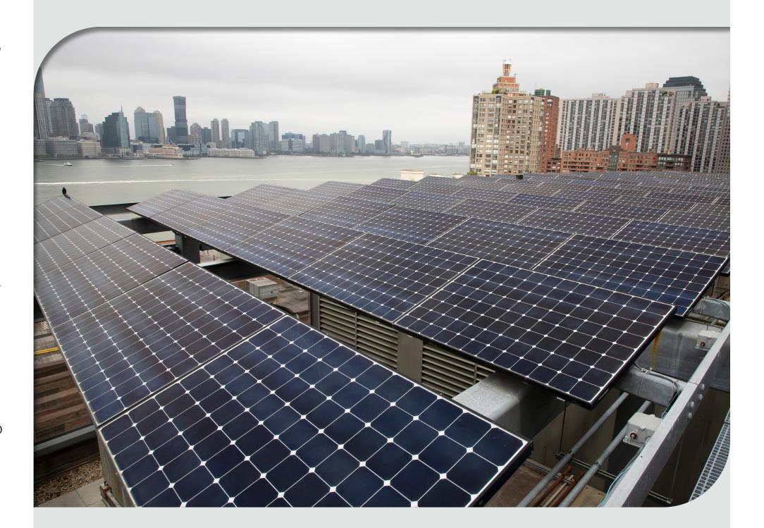
Solar panel installation on the roof of the Battery Park School in lower Manhattan. In FY22, DCAS installed 10 solar panel systems like this one in schools across New York City, adding three megawatts of solar capacity to the City's portfolio, a 23% increase from the previous year.
