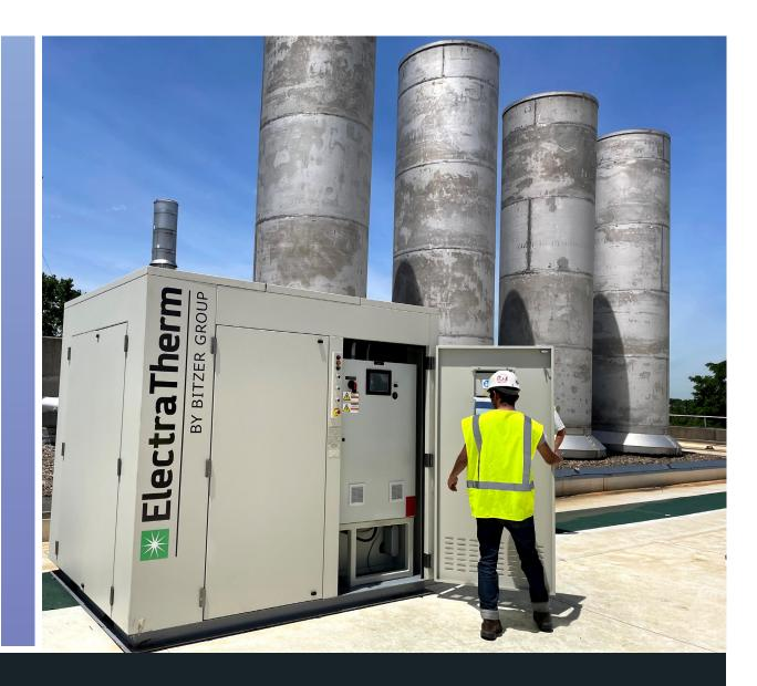
DCAS staff inspecting a recently installed new technology project as part of DCAS's Innovative Demonstrations for Energy Adaptability (IDEA) program. This installation captures waste heat and generates electricity.
