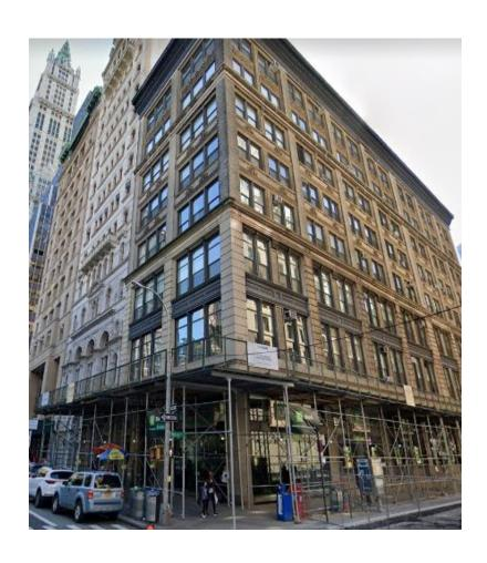
Mesh parapet for required for sheds installed under 2022 Code:
