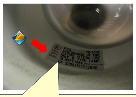
"Other fixtures" will generally be screw-based luminaires (compact fluorescent, tungsten/halogen, or incandescent). For LEDs, total draw can be deceptive – assume the maximum wattage listed on the luminaire.
