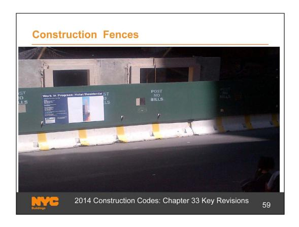
Construction fences must: be painted Hunter Green; have the Construction Information Panel installed; have 12" square viewing panels every 25 feet; and have no other construction-related signs or messaging (including "Post No Bills) affixed.
